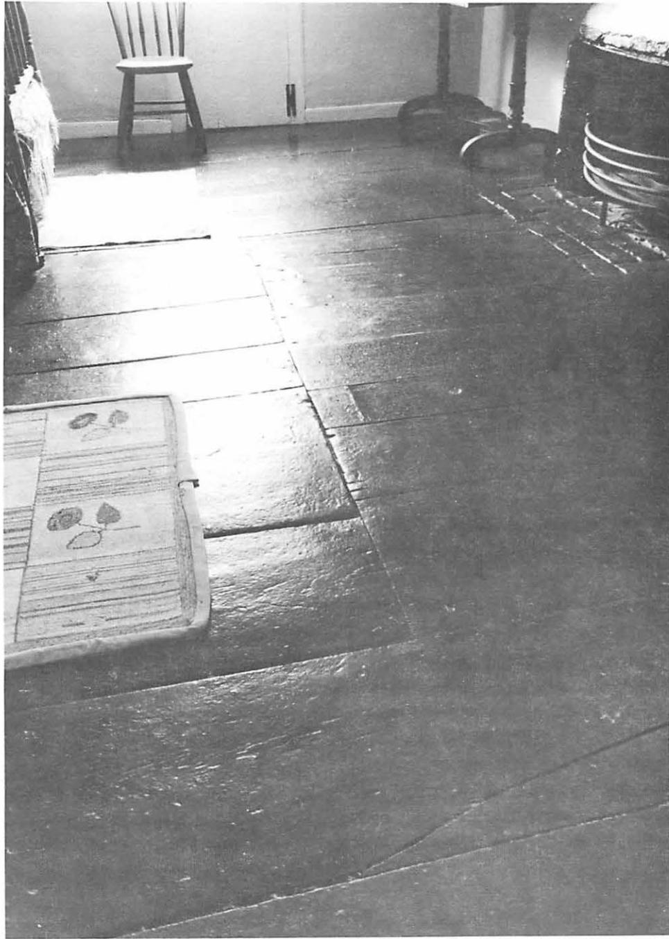
The joints in the floor boards show where the original 1767 kitchen fireplace chimney was removed. In 1781 it was rebuilt the other side of the original end wall, allowing the fireplace to merely penetrate the wall, and so provide a larger bedroom.
