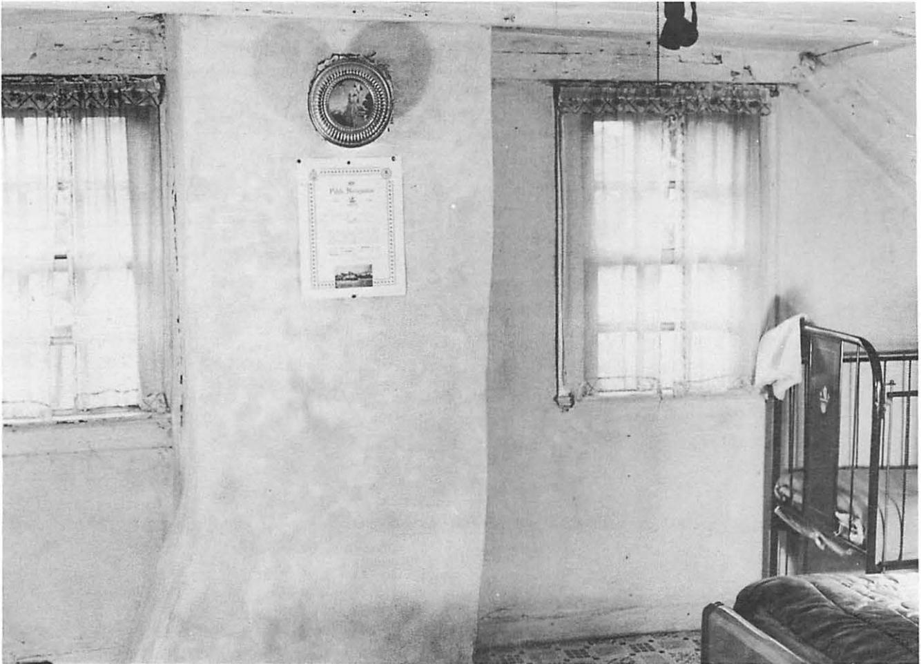
Bedroom 1. Photograph of 1947. A cap over the stove pipe connection is a reminder that Simeon Perkins poured water in here to douse a chimney fire started in the office below. This is only possible because the three fireplaces shared a common flue.
