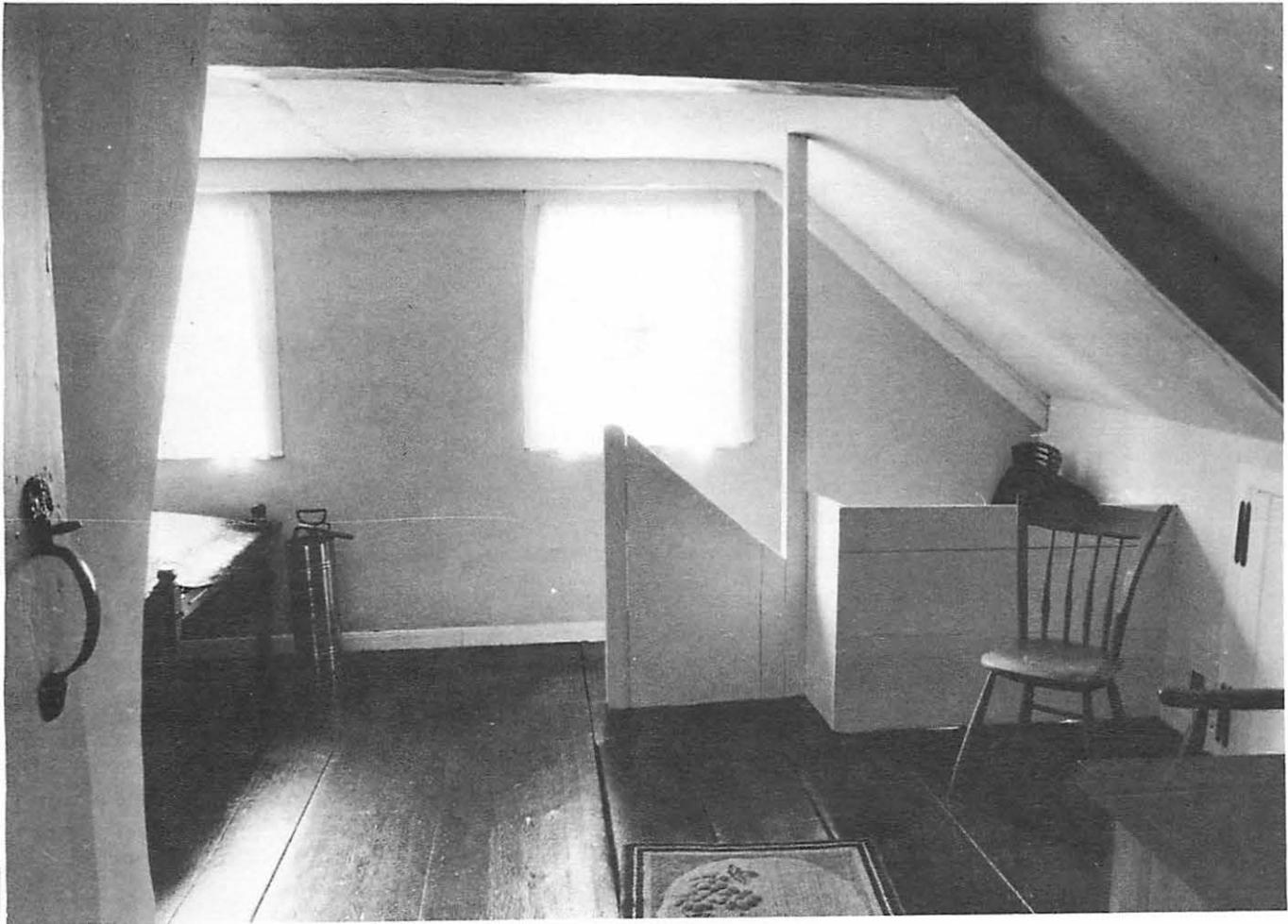
Bedroom 3 looking east. Marks in the end wall and ceiling suggest a partition has been removed, which would have divided this room into two rooms, each with a window.
