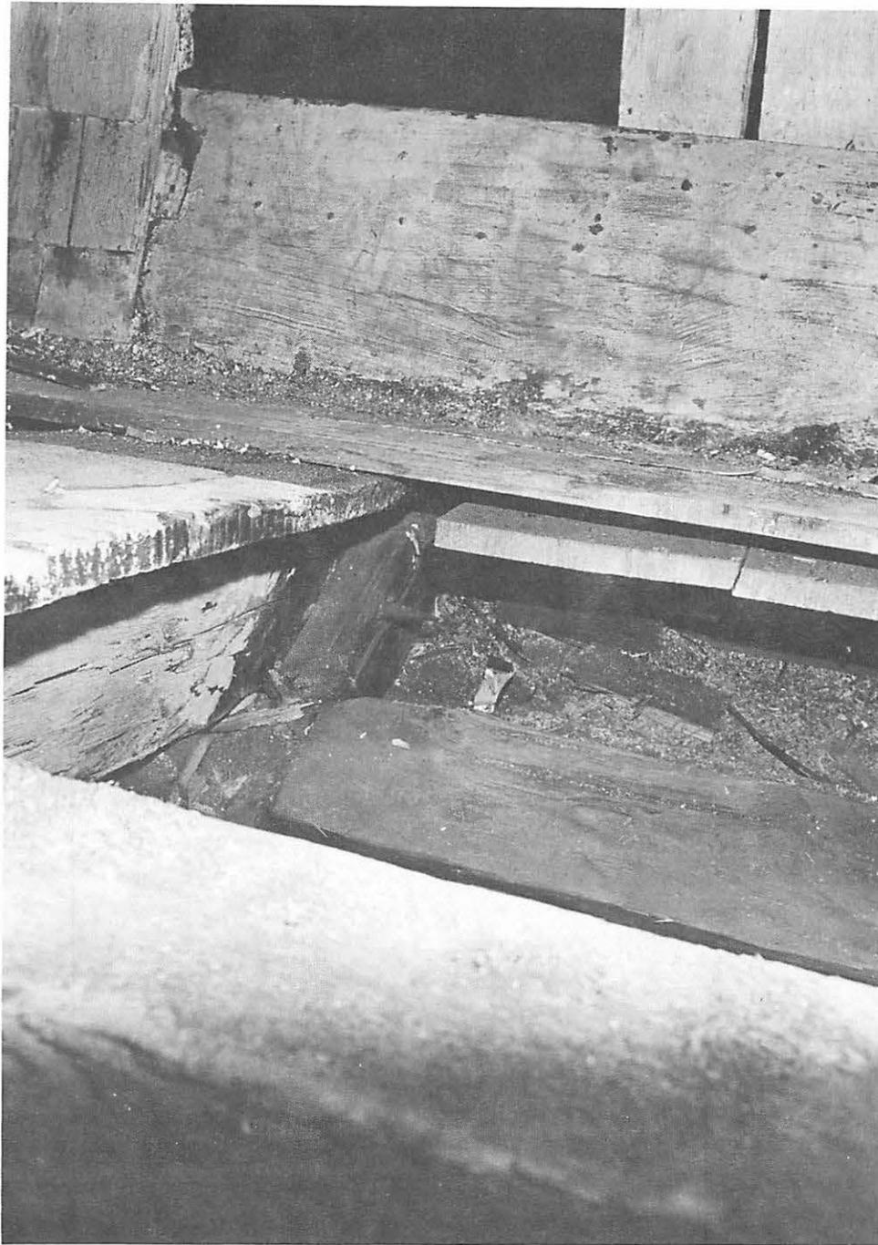
Kitchen Attic looking down on the original valley gutter of 1792. At the middle left can be seen the tree-nail at the joint between the rafter and horizontal tie beam which acts as a floor joist. In the immediate foreground is a purlin. The hole at the top leads into the attic roof space over the kitchen. This space is beyond the reach of visitors. At the top left are the 1792 shingles.
