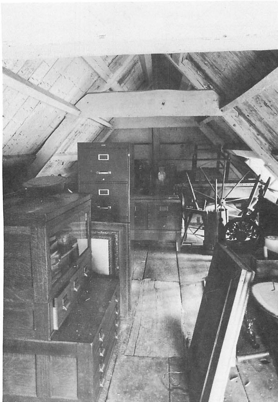
The Kitchen Attic looking north. Note the low dormer window height and the high roof space. At the far end is the 1792 roof slope with horizontal boarding. In the foreground can be seen the patch in the flooring where the brick flue was located prior to 1949. Substantial reconstruction of the roof has taken place as modern purlins and boarding show.
