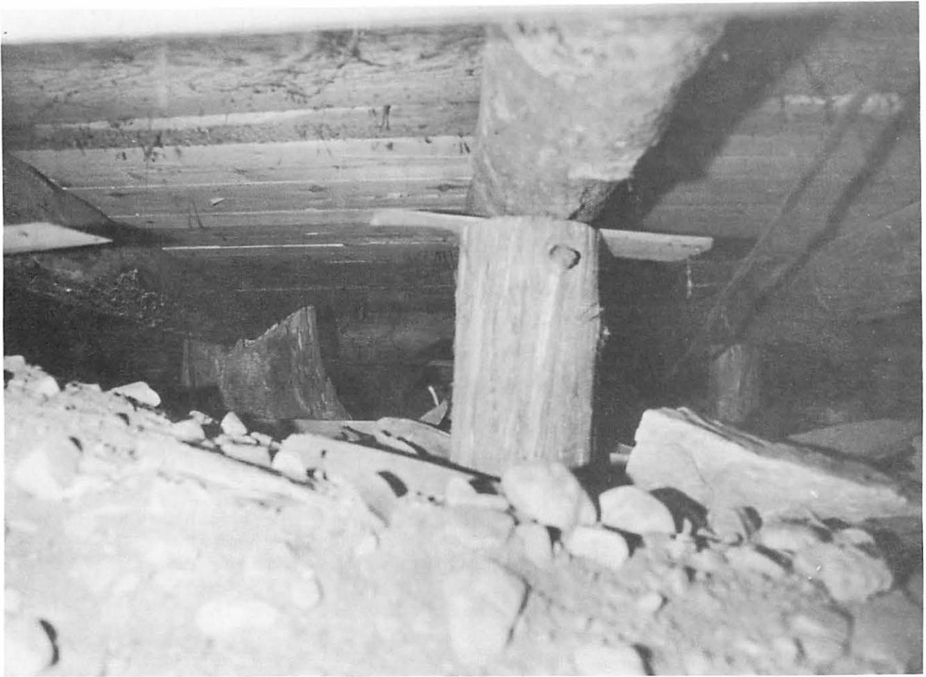
The Cellar looking west under the parlour floor. The new floor supports were installed in 1949. What appears to be a tree stump, left centre, may really be one! If so, it supports the theory that speed of construction was important, and no time or expense was wasted on grubbing out tree roots.
