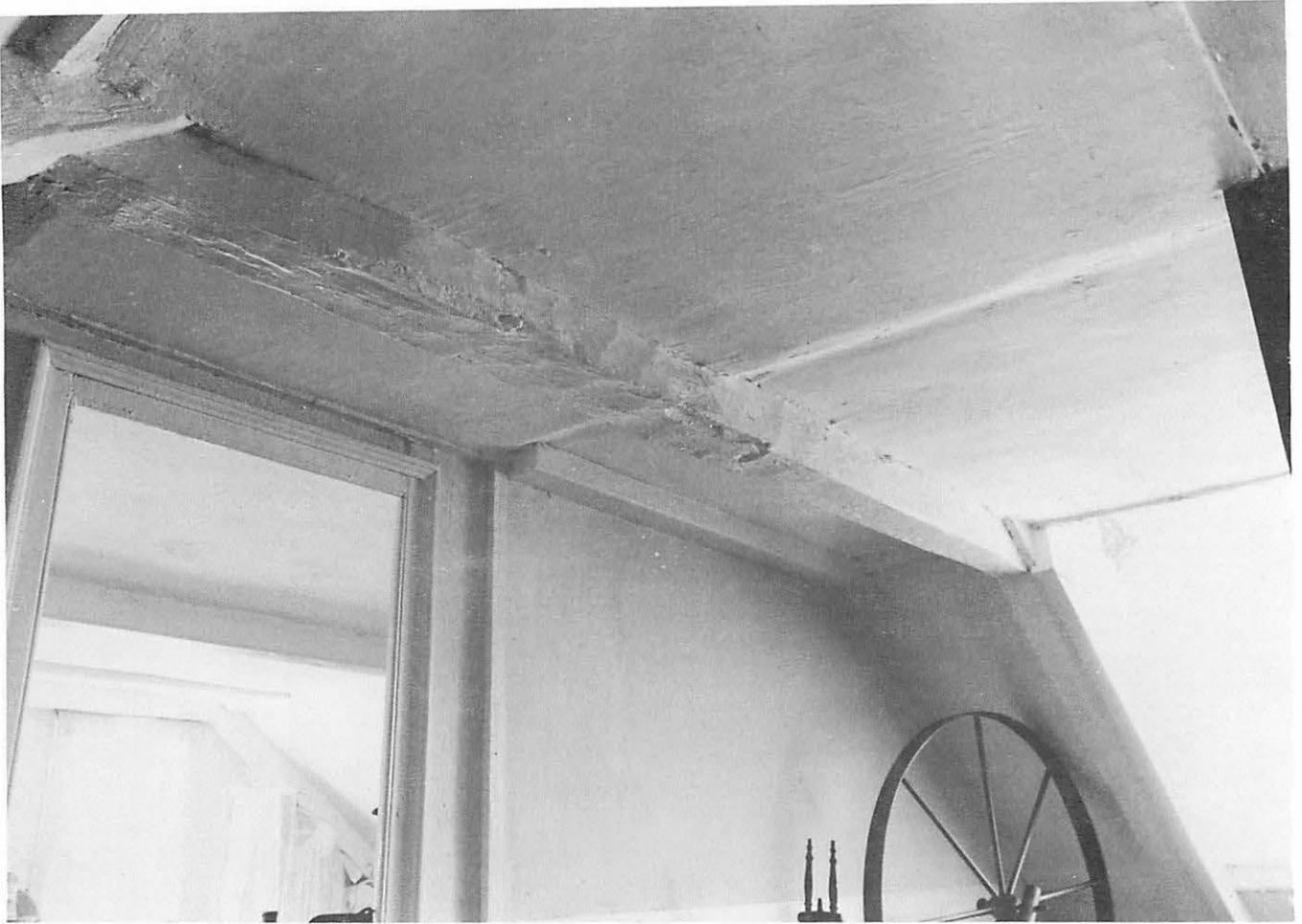
The Stair Landing ceiling 1979. Some traces of change can be plainly seen in the plaster ceiling, while others, for example an access hatch, have been hidden by it. The marks of the adze can be clearly seen in the ceiling beam.
