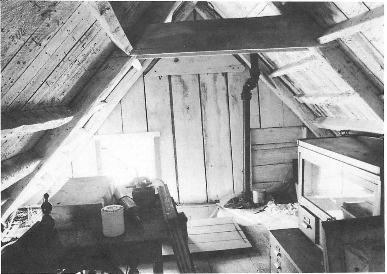
The Kitchen Attic looking south. Note the second south facing window, which has been filled in to the right, and the low window height.
