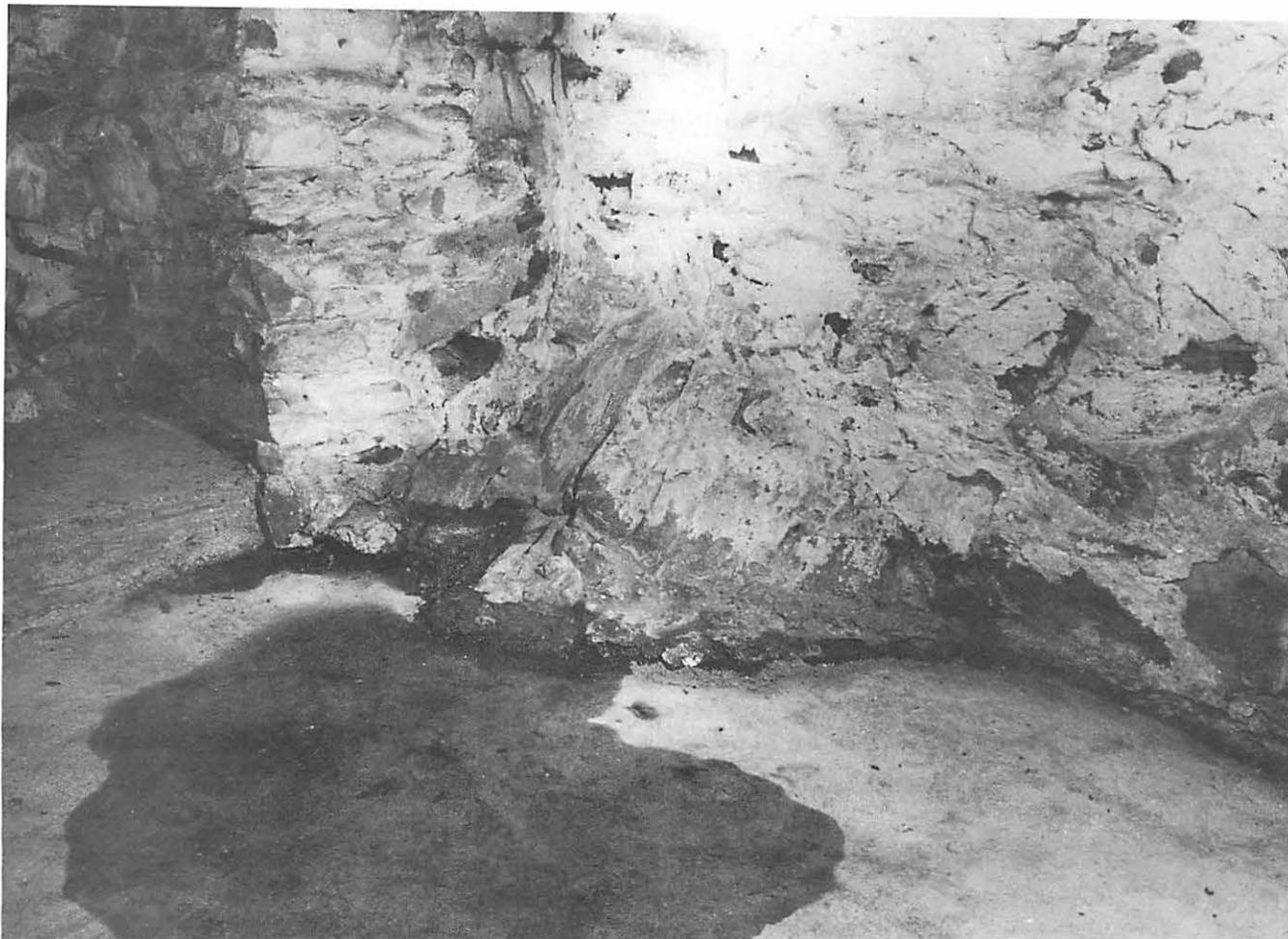
The Cellar. The stone outcrop seen in the southwest corner may be part of the reason for limiting the cellar size. A concrete floor was installed in 1949. Access is to the left.
