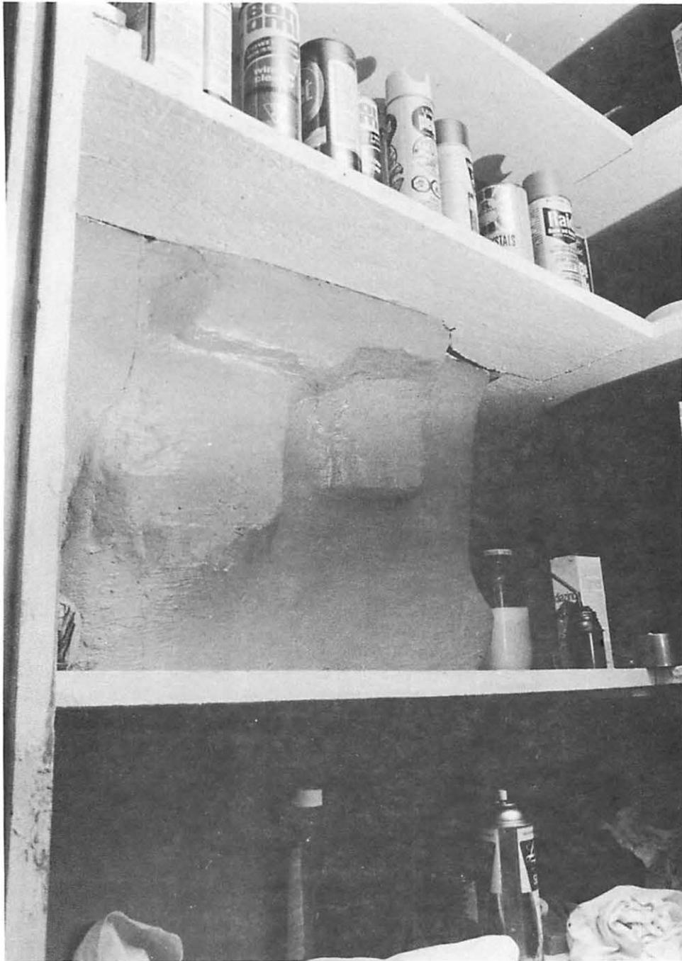
The Kitchen. In the closet to the right of the fireplace the remains of a brick oven can be seen. The oven was removed on April 28, 1800, to form this closet.
