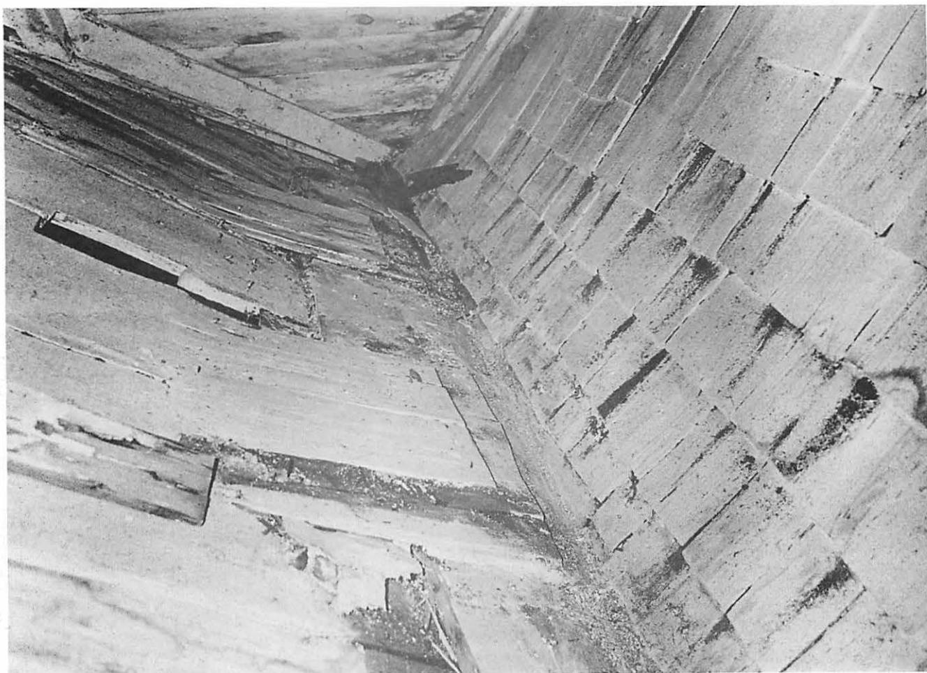
The Roof Junction. The original roof can be seen on the left with some shingles still in place at the bottom of the slope. As these are above the valley gutter, the shingles themselves must date from 1792. The shingled roof of 1792 is on the right. The surfaces have been whitewashed at some time.
