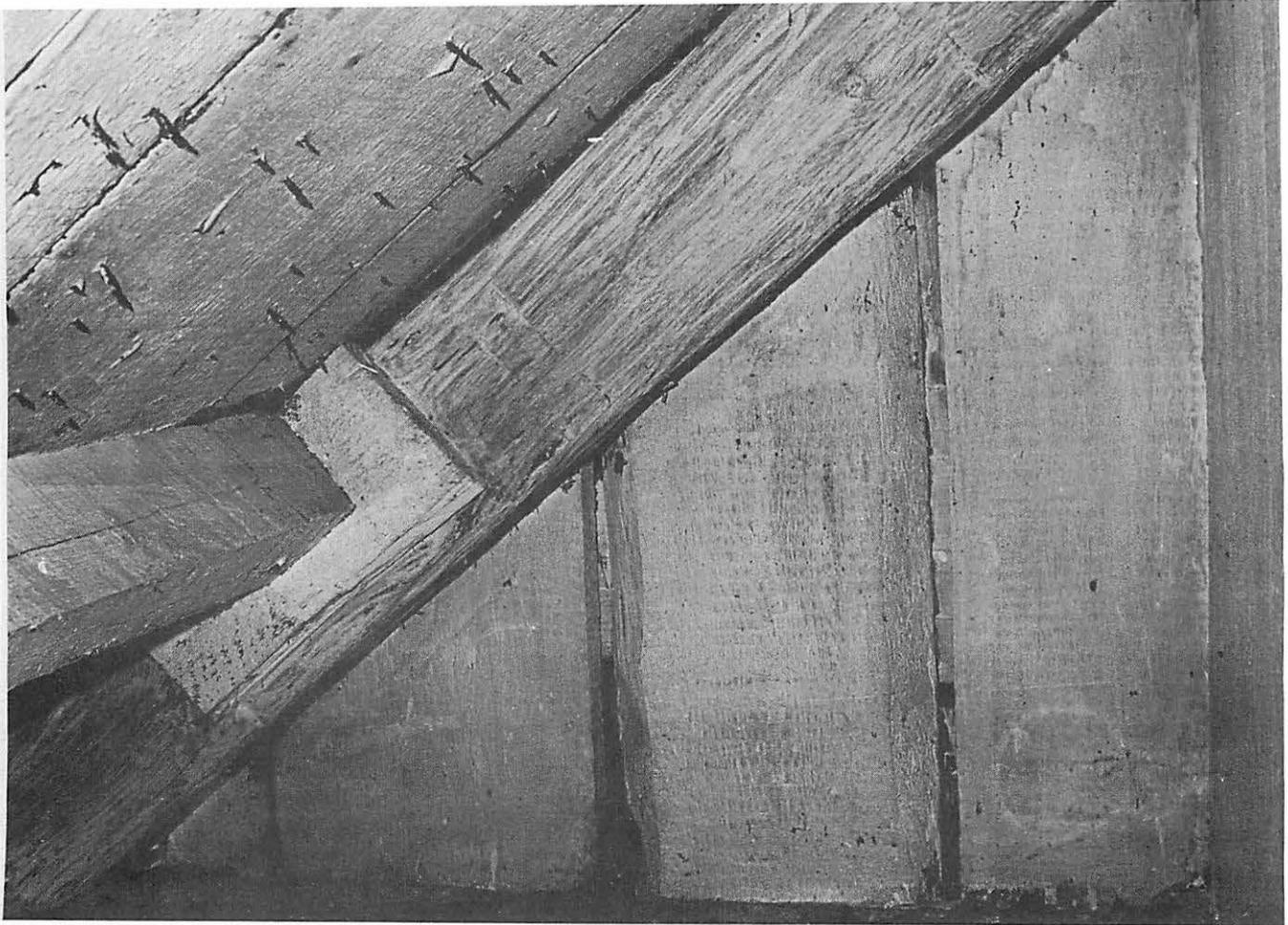
Bedroom 2 Closet. The inside of the original 1767 gable wall shows no sign of birch bark or other draught-proofing materials behind the clapboards. The vertical boards clearly show the saw marks from the water powered saw mill, whereas the rafter shows the less regular surface of the adze or broad axe. The purlin on the left is recent, from 1935 or from 1949.
