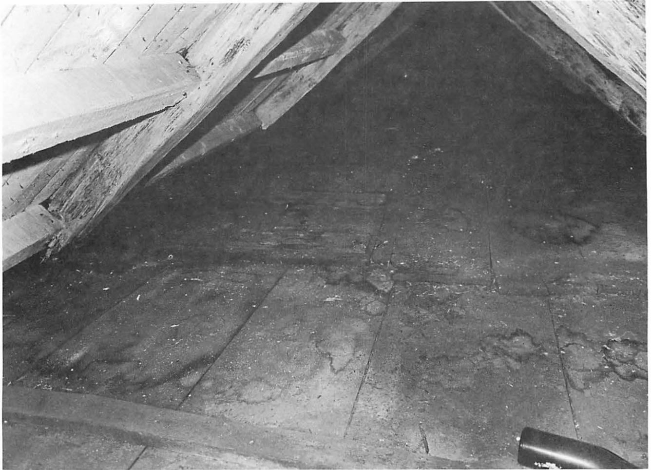
The Attic. At the middle-left can be seen the top of the access hatch which has been plastered over at some time on the ceiling below. The purlins and boarding on the left-hand roofslope date from 1935.
