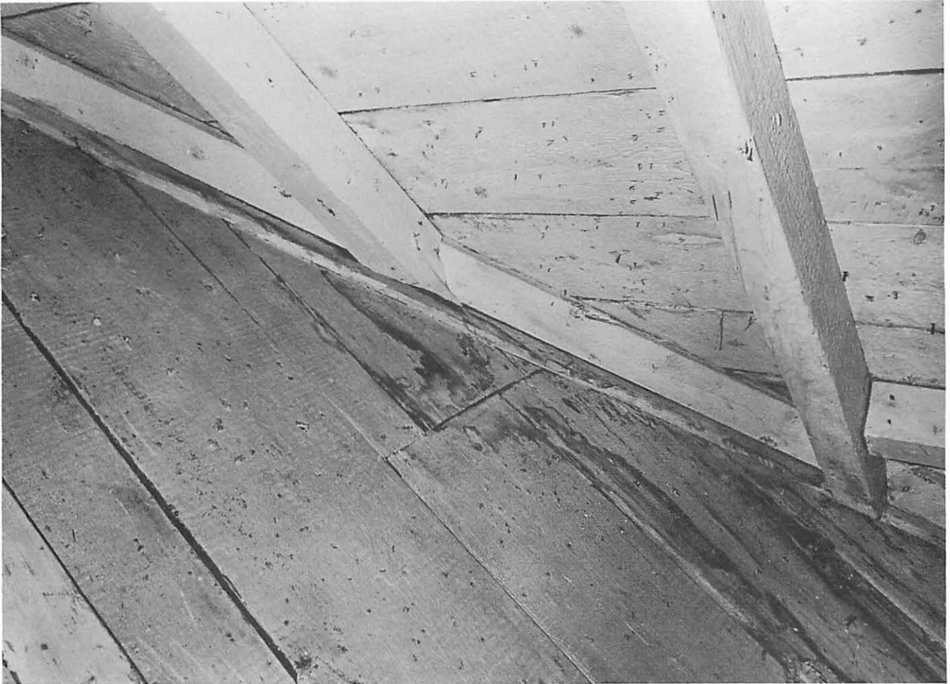
The Kitchen Attic. At the bottom is the original roof sheathing. In the centre is the break in the boards where the dormer was located until after 1792. At the top is the infill roofing, with horizontal boards possibly installed around 1840.
