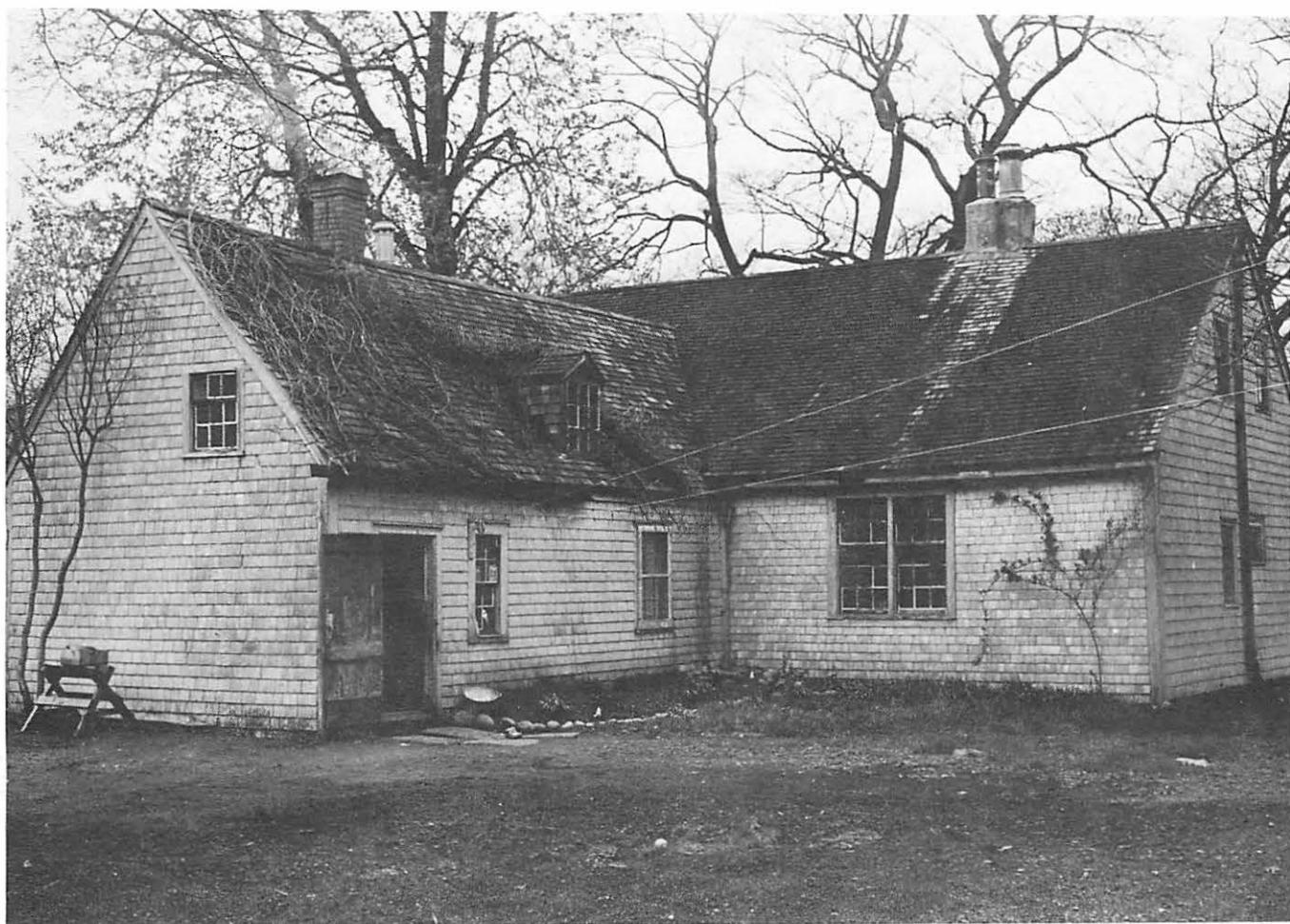
View from the southeast. This photograph was taken in 1947 before any repairs were carried out by the Province, but shows the state of the roof where it was repaired in 1935. Note the lack of window putty and paint. At the right-hand end can be seen the vent pipe from the plumbing installed this century. Victorian chimney pots and a stove chimney can be seen. The banked up soil and creeper on the roof provide clues to causes of rot.
