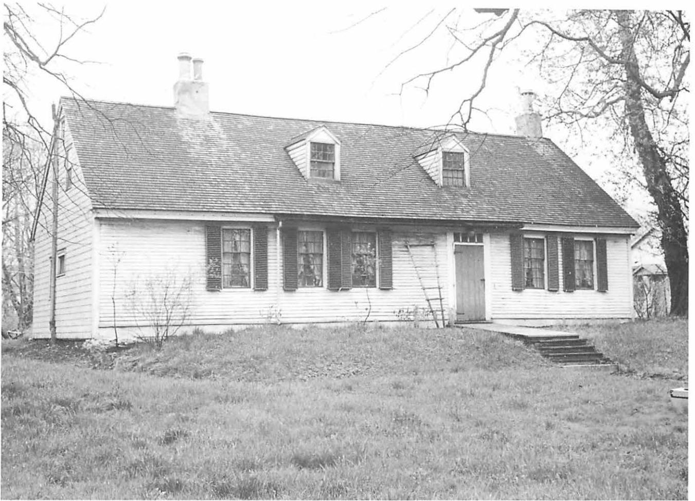
The north front in 1947. Note the horizontal window and plumbing stack on the east end, (left hand side) and the Victorian Gothic Chimney Pots. The overall deformation of the house can be seen by the drooping ends.
