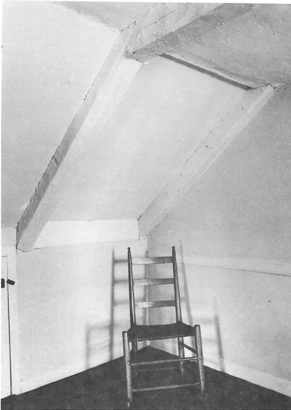
Bedroom 2. The filled-in dormer window in the southwest corner. Not required until after 1781, when the end windows would have been blocked by the addition, the dormer was in use after 1792 when the kitchen wing was added. It is not known when it was removed but presumably it could have been taken out when the stair was altered about 1840.
