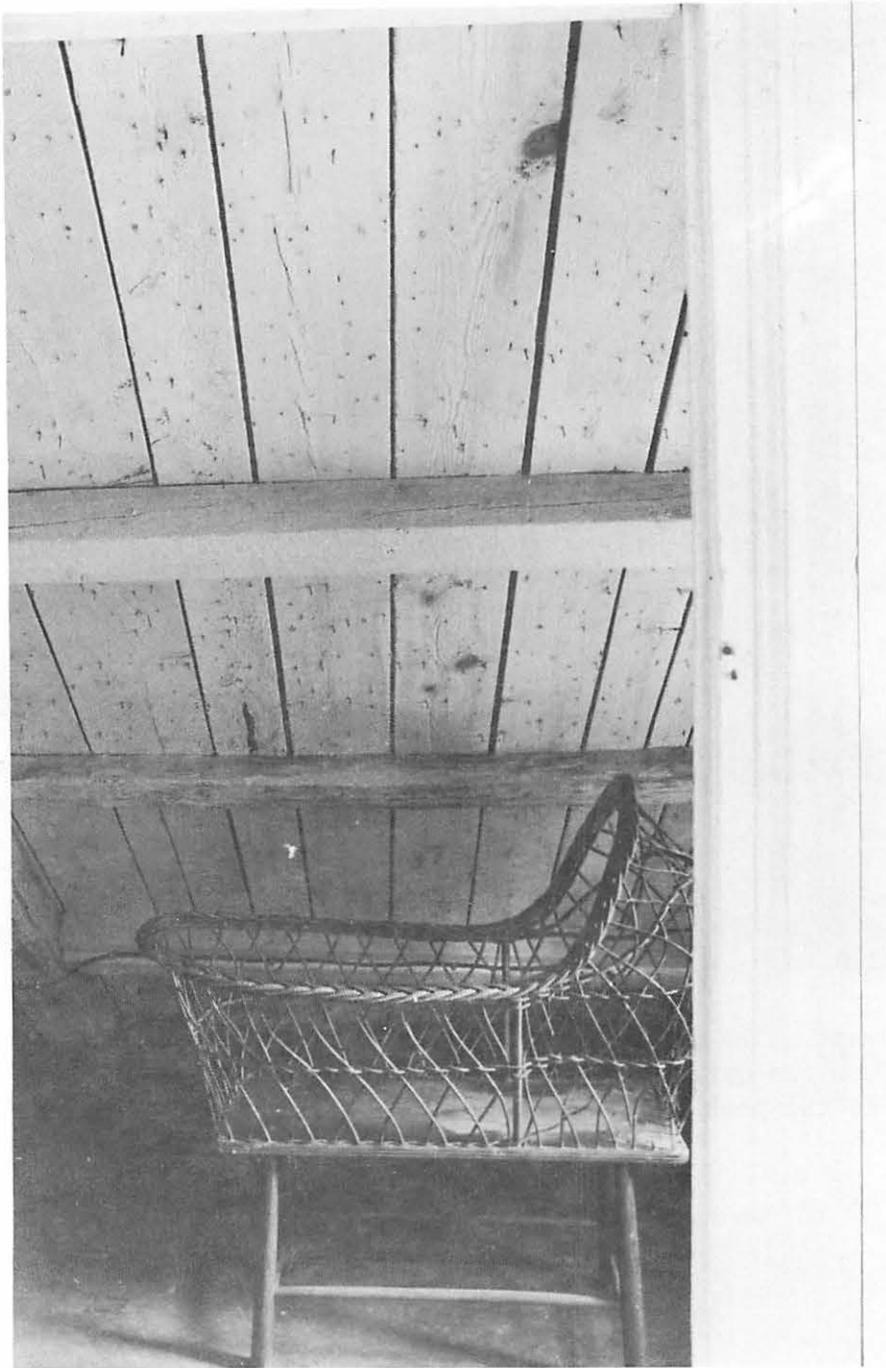
Bedroom 1 Closet looking south. The horizontal purlins spanning between the rafters and vertical boarding can be clearly seen through the open doorway. In contrast to the original boards, those used in 1935 are much narrower. See next photograph.
