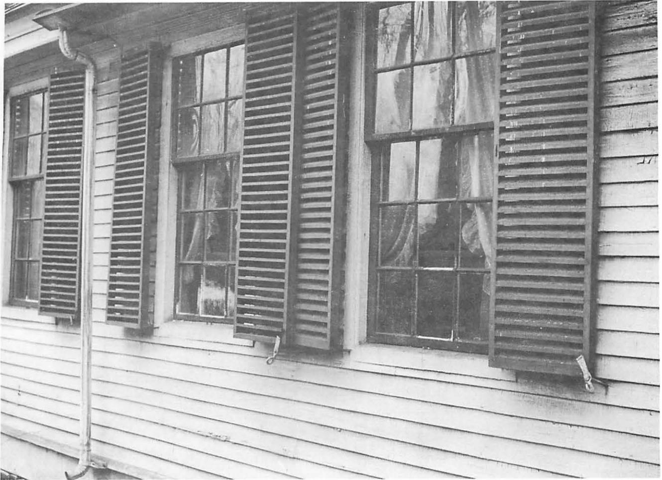
Part of the North front photographed in 1947, which clearly shows the sag at the left hand end due to the rotting of the timber sills. The original house ended at about the position of the Rainwater pipe as can be seen in the change in the roof shingles, The right hand shutters have been installed upside-down.
