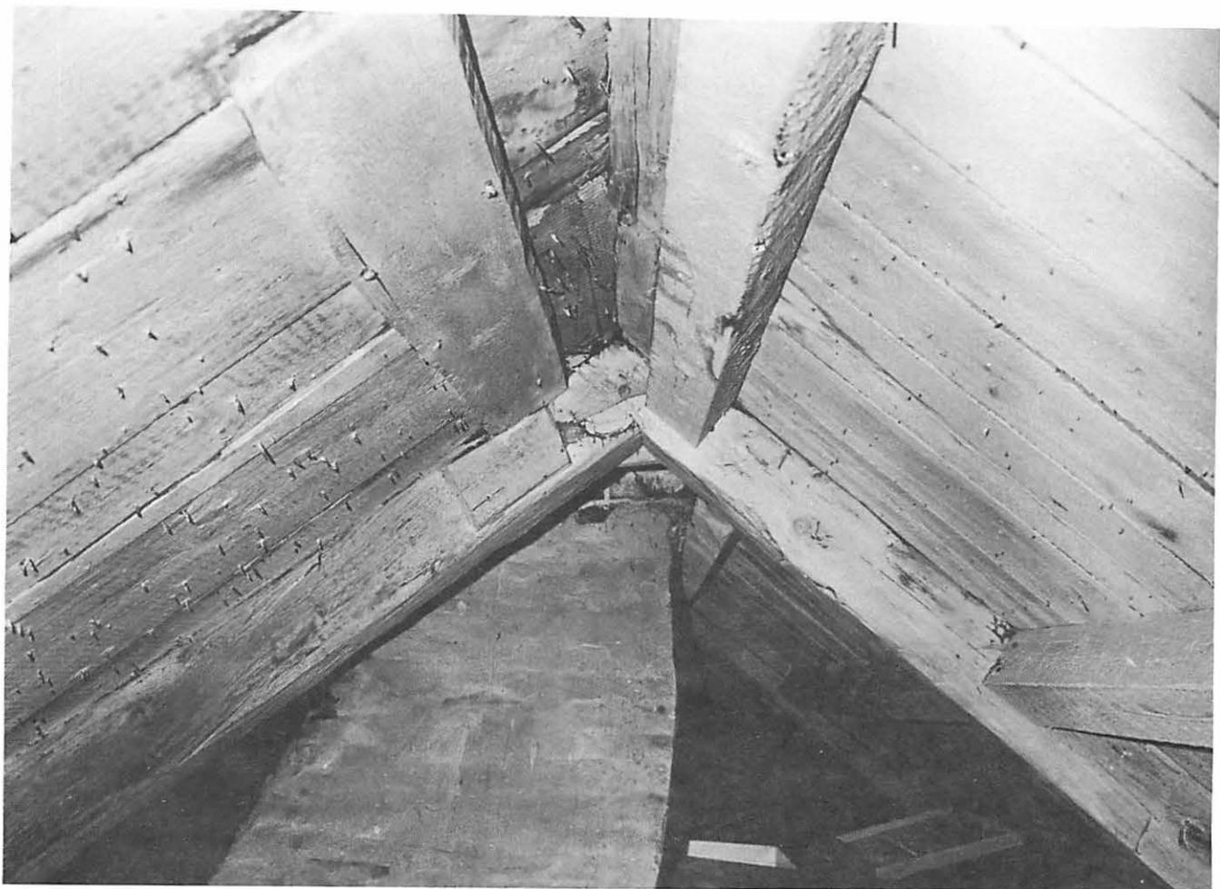
The Attic. At the top centre can be seen the position of the chimney up until its removal in 1781, when it was relocated beyond the original end frame in the new extension. Because the planking on the roof slope to the right was replaced in 1935 the visible clues occur only on the left-hand (north) roofslope.
