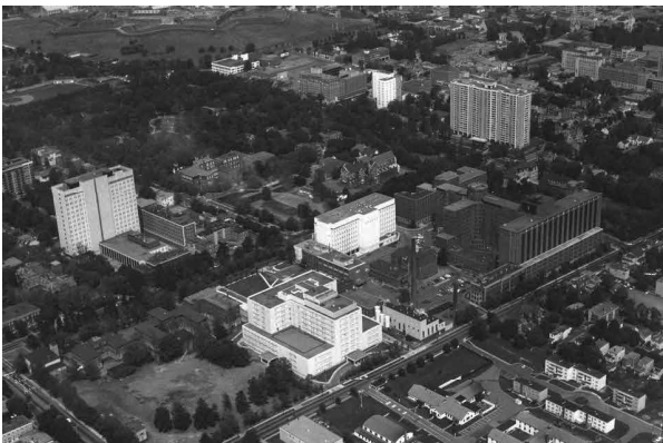
Figure 2. Aerial photograph of IWK Children's Hospital. The original Grace Maternity Hospital is seen, as well as the Victoria General Hospital's "Jubilee Building," demolished in 1980 to make way for the Robert Clark Dickson Ambulatory Care Centre. ca. 1972. Courtesy of the Dalhousie University Photograph Collection, Dalhousie University Archives, Halifax, Nova Scotia.
