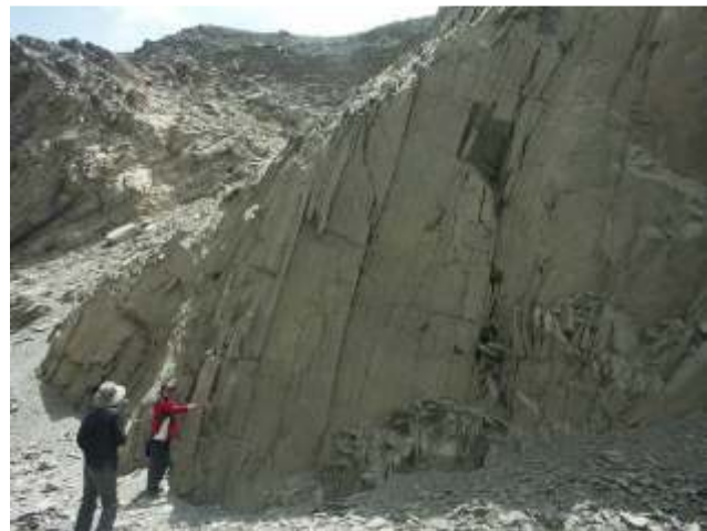
Fig. 2 Buckling failure of rock bedded slope in K765
