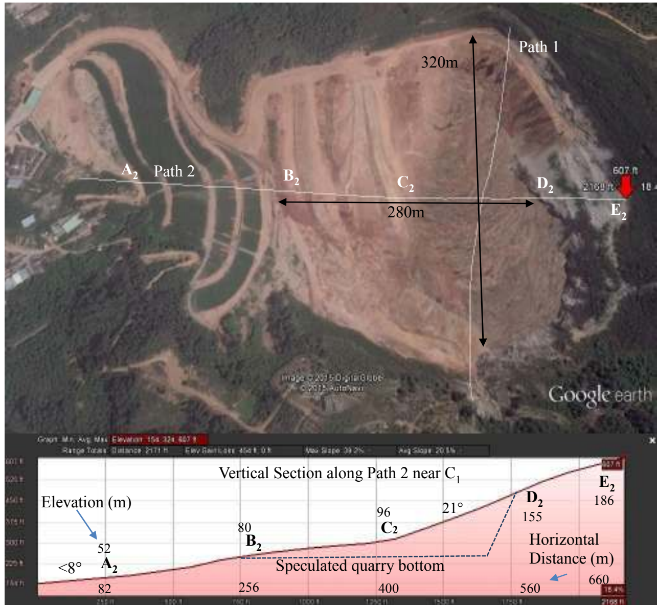
Fig. 4 Section view Path 2 (Google earth image facing East, Oct. 2015). Average slope between C 2 and D 2 on different sections varies between 21° ~ 27°, with max slope of 45° ~ 49°. Elevation at the industrial park is approximately 30 m.
