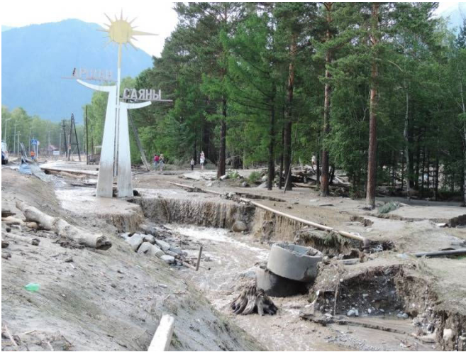
Figure 6. Ravine formed by water flow along the Traktovaya street near the “Sayany” resort. Picture of June 28, 2014. Local time 18:30 (point 790 – 51°54'03.5", 102°26'43.3")
