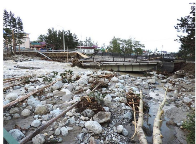
Figure 12. Bridge over the river Kyngarga on June 28, 2014, after the passage of debris flood along the river. Local time 19:18. Photo from the right bank of the river (point 674 – 51°54'51.7", 102°25'36.4")
