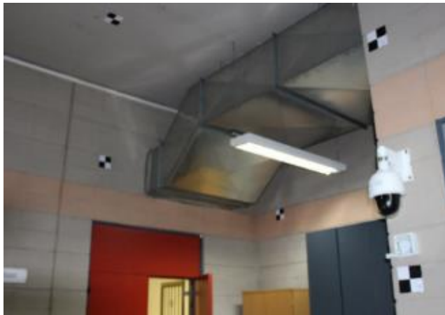
(b) The concrete wall
