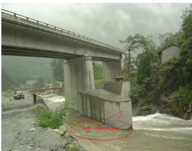
Fig. 11 The anti-collision pier applied for Den Jigou bridge pier protection
