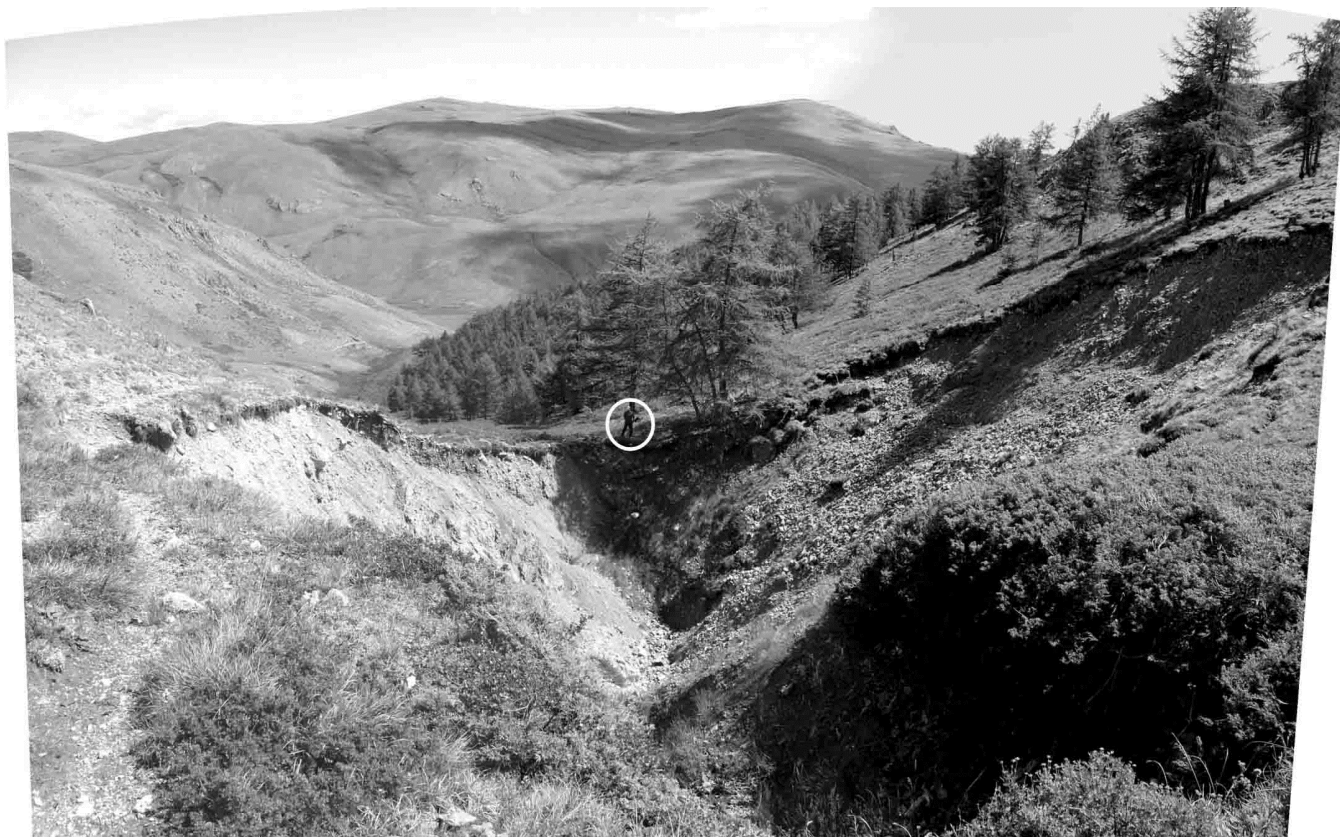
Figure 4. Ground subsidence in Riphean-Vendian marbled limestones in the central part of the Chagan-Uzun massif. Person in a circle is 1.8 m tall
