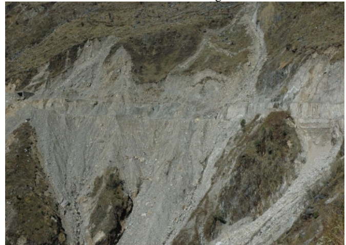
Plate 4. Andha bridge slide along Gangtok-Nathula road (2007)
