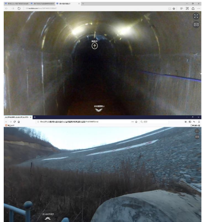
Figure 9 3D panoramic image of flood culvert entrance
