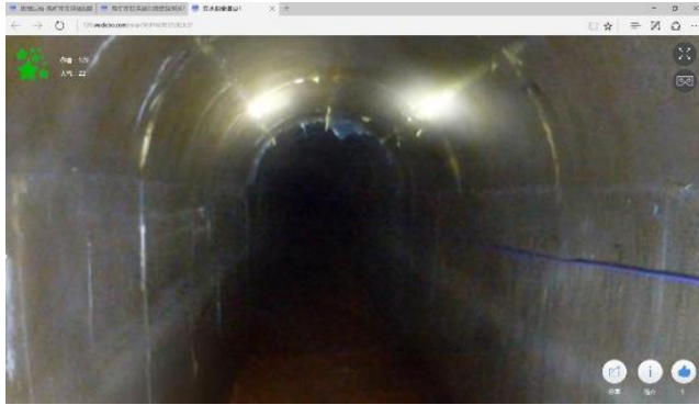
Figure 8 3D panoramic image of tailings dam drainage tunnel
