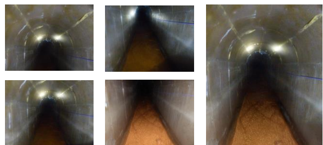
Figure 7 Flood culvert 3D panoramic image of tailings dam drainage tunnel
