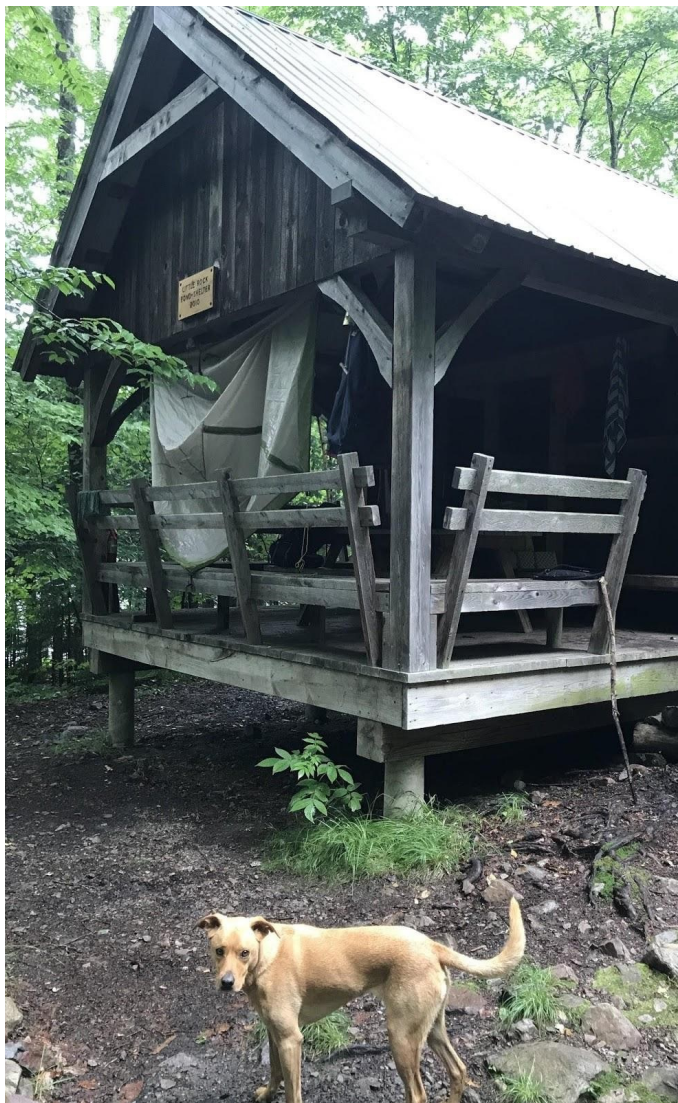
Figure 2. Little Rock Pond Shelter on the AT/LT
