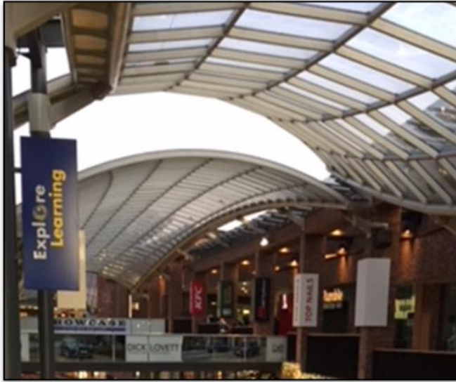
Figure 1: Cabot Circus roof [Photo by author]
