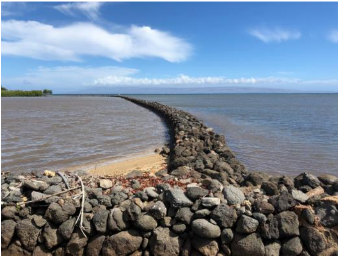
Figure 1 - Kuapā (walls) built using the traditional dry-stack method on Moloka'i. Photo by Evelyn Cornwell.
