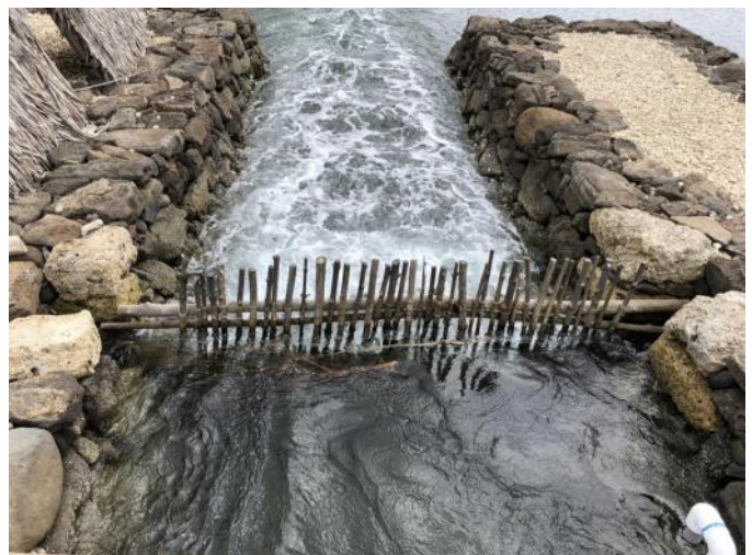
Figure 2 – Channel with mākāhā (sluice gate) leading into fishpond A from the ocean at high tide. Photo by Evelyn Cornwell.
