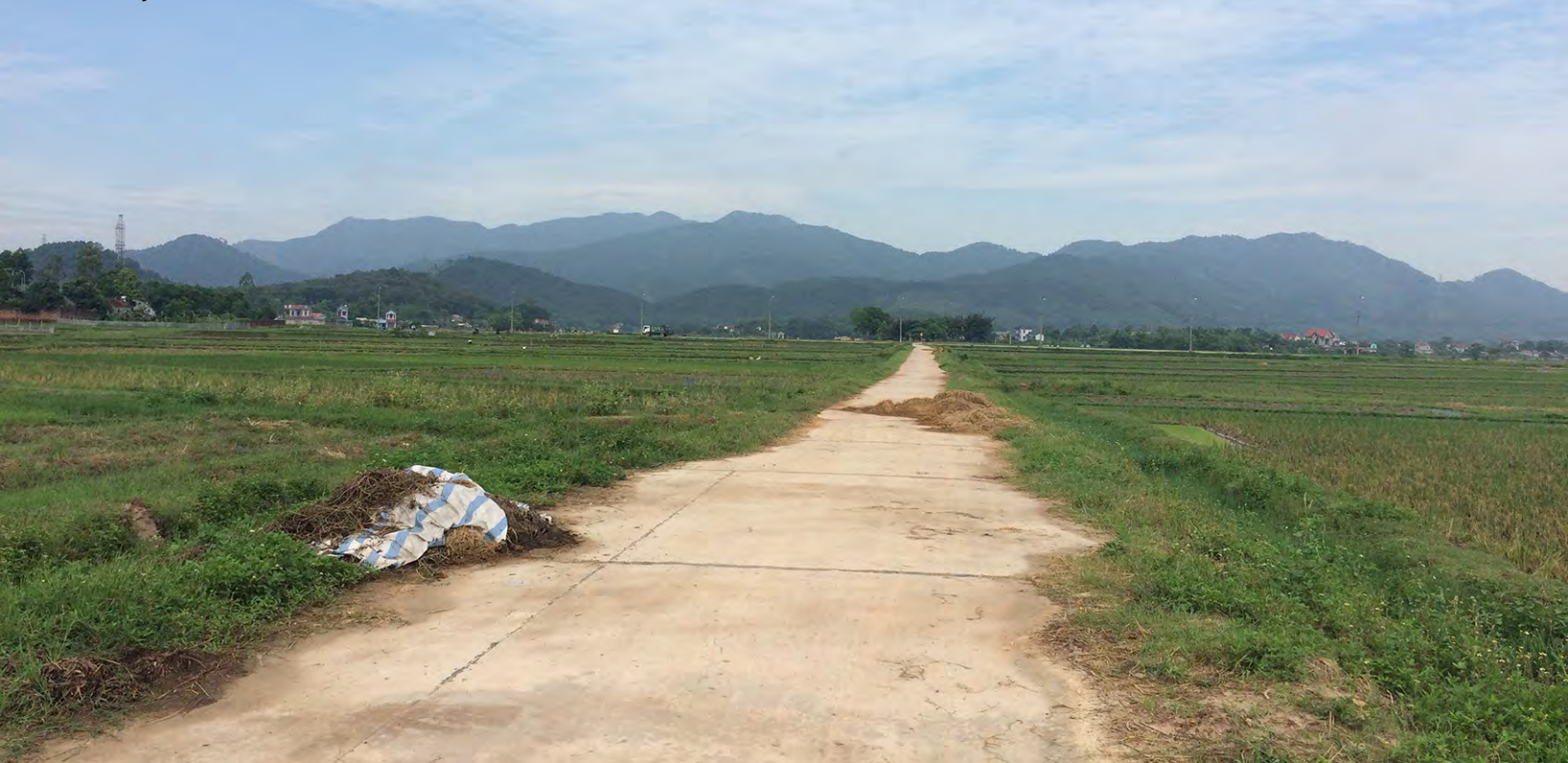
Figure 6: Asphalted road. Photo by author.
