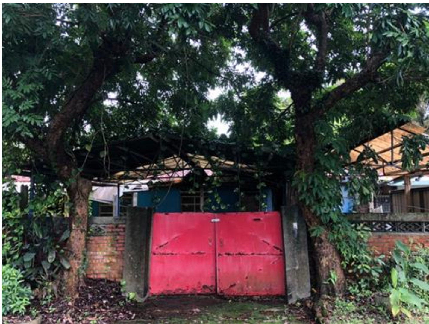
Figure 7: Abandoned house in Zhong Xing New Village. Source: Photo by author, 2019
