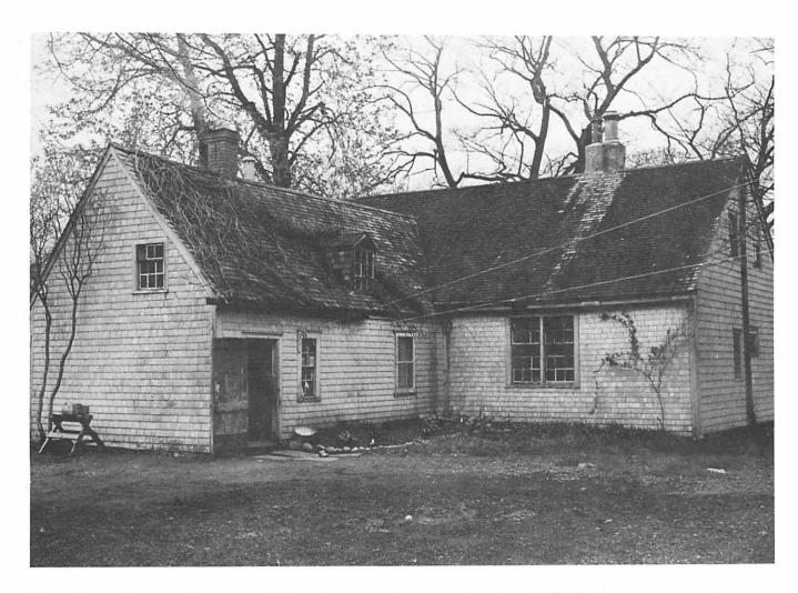
View from the southeast. This photograph was taken in 1947 before any repairs were carried out by the Province, but shows the state of the roof where it was repaired in 1935. Note the lack of window putty and paint. At the right-hand end can be seen the vent pipe from the plumbing installed this century. Victorian chimney pots and a stove chimney can be seen. The banked up soil and creeper on the roof provide clues to causes of rot.
