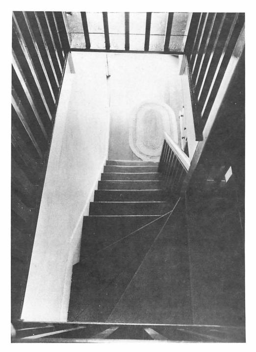
The Stairs looking down. Built in 1949, the design of the staircase repeats the dimension of that believed to have been built in 1766 and removed about 1840.
