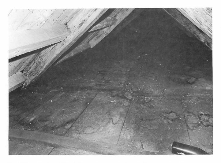
The Attic. At the middle-left can be seen the top of the access hatch which has been plastered over at some time on the ceiling below. The purlins and boarding on the left-hand roofslope date from 1935.
