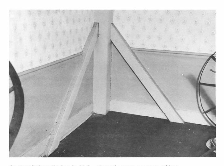
The Ground Floor Chamber in 1947. Diagonal braces are very evident in the extension of 1781. The extremely thin perimeter wall can be imagined as the brace is not hidden within it. The wall is only 150 mm thick.
