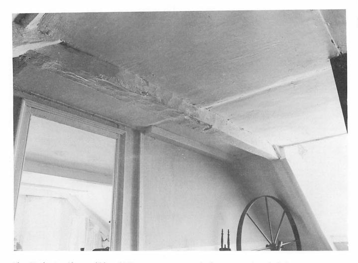
The Stair Landing ceiling 1979. Some traces of change can be plainly seen in the plaster ceiling, while others, for example an access hatch, have been hidden by it. The marks of the adze can be clearly seen in the ceiling beam.
