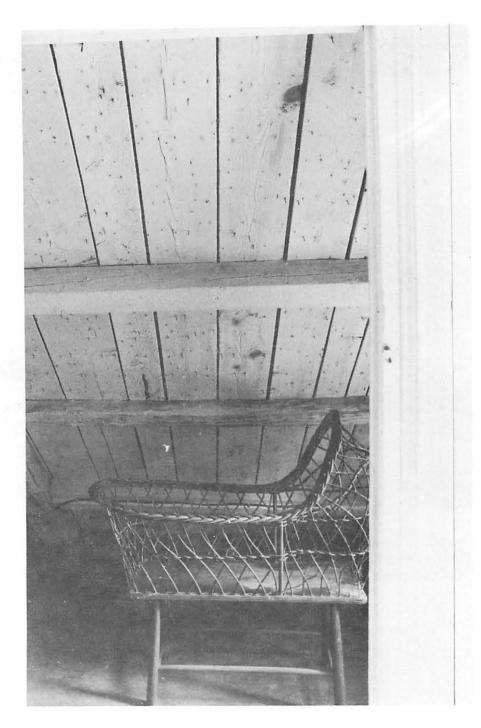
Bedroom 1 Closet looking south. The horizontal purlins spanning between the rafters and vertical boarding can be clearly seen through the open doorway. In contrast to the original boards, those used in 1935 are much narrower. See next photograph.
