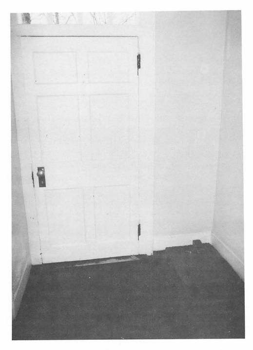
The inside of the front door in the north wall. The lock has been changed at least twice and rising-butt hinges installed, but the door appears to be either original or at least early. To the right of the door can be seen bolts with large squre washers supporting the commemorative plaque on the outside.
