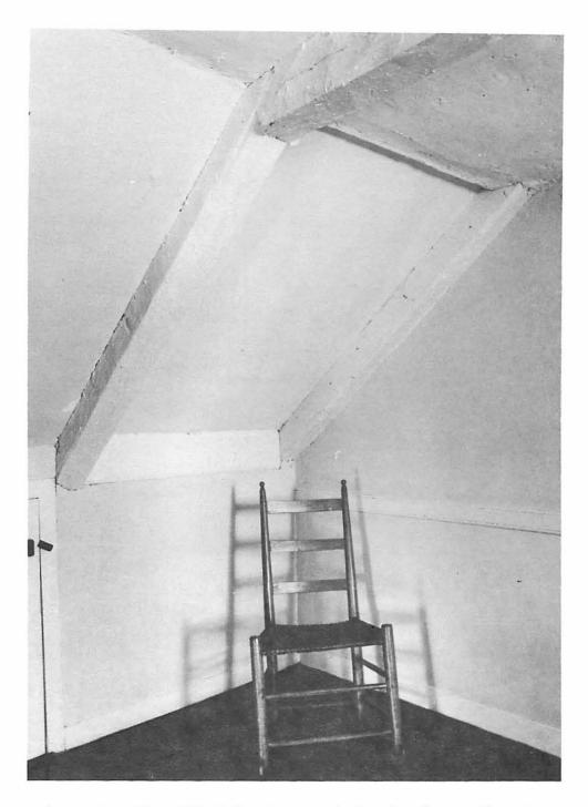
Bedroom 2. The filled-in dormer window in the southwest corner. Not required until after 1781, when the end windows would have been blocked by the addition, the dormer was in use after 1792 when the kitchen wing was added. It is not know, when it was removed but presumably it could have been taken out when the stair was altered about 1840.
