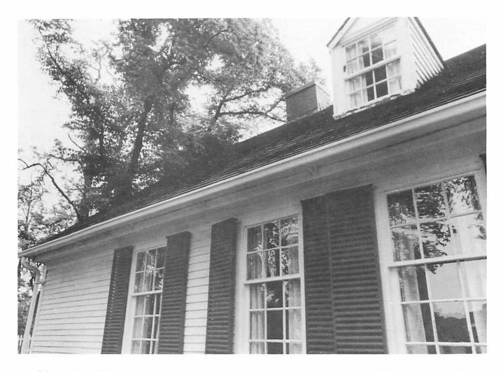
Junction of addition and original house. The extent of the addition can be clearly seen by the hump in the roof which locates the original end wall.
