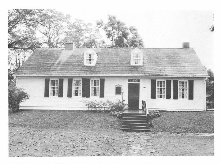
The North Front in 1978. The lack of symmetry is caused by the addition to the left hand end in 1781 and the later dormers.
