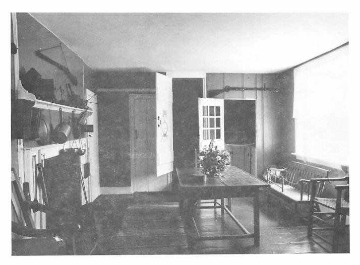
The Kitchen looking east. This end of the room was altered by the addition of the stair in 1782. As storage is integral with the stair, it would appear that the pantry was built at this time as well.
