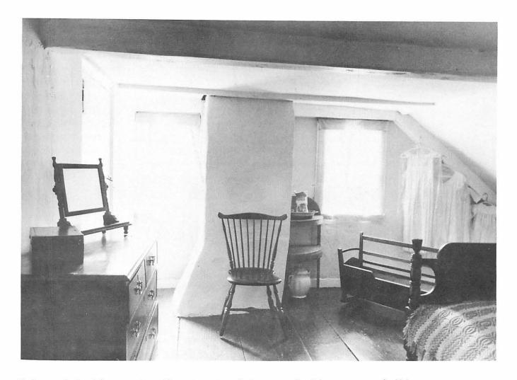
Bedroom 1 looking west. The structural frame and chimney are visible with the 2 flues from the Office and Parlour gathering into one to eject smoke close to the peak of the roof.
