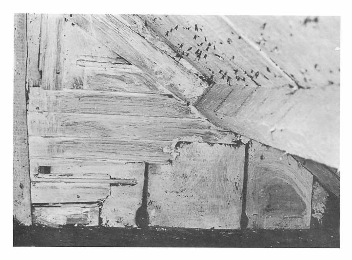
Bedroom 3. Clapboarded gable wall from 1767. This is definitely original as it was left untouched when the 1781 addition covered it over. The vertical boarded wall can be seen with mice holes gnawed at floor level. These original clapboards match those on the front or north elevation which supports the idea that the front is still the original cladding.
