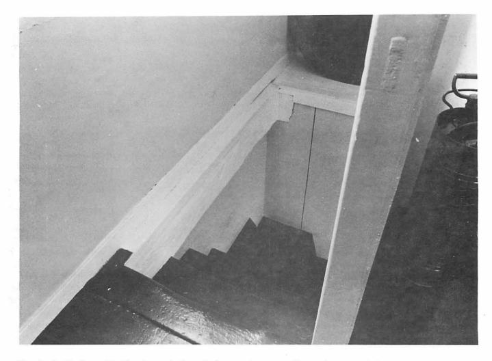
The Back Stair. At the top of the stair can be seen the cut-away girt or end beam to ease access to the kitchen below. The room above is called a 'Garret' in the Diary and the narrow stair fits that image.
