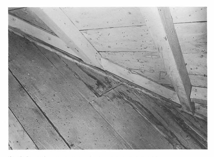
The Kitchen Attic. At the bottom is the original roof sheathing. In the centre is the break in the boards where the dormer was located until after 1792. At the top is the infill roofing, with horizontal boards possibly installed around 1840.
