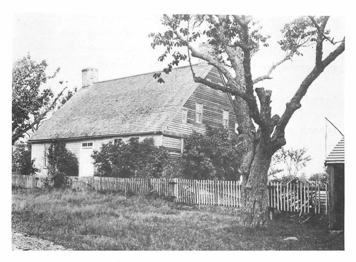
The Lane House, Killingworth, Connecticut. Note that the gable end projects slightly over the end wall, there are two chimneys, one at each end of the ridge, and the front is symmetrical. The house is clapboarded.
