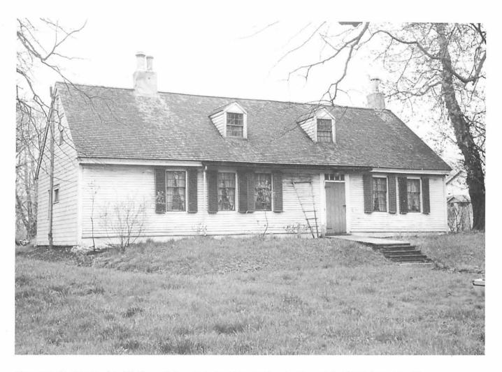
The north front in 1947. Note the horizontal window and plumbing stack on the east end, (left hand side) and the Victorian Gothic Chimney Pots. The overall deformation of the house can be seen by the drooping ends.
