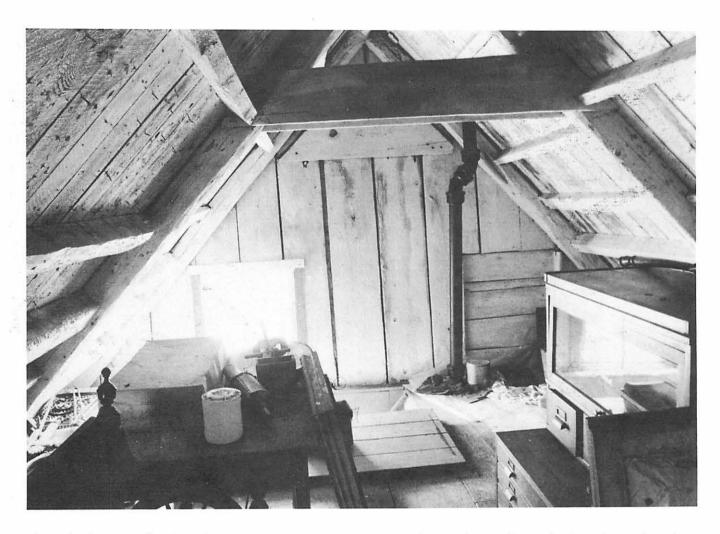
The Kitchen Attic looking south. Note the second south facing window, which has been filled in to the right, and the low window height.
