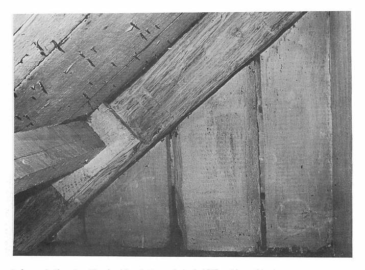
Bedroom 2 Closet. The inside of the original 1767 gable wall shows no sign of birch bark or other draught-proofing materials behind the clapboards. The vertical boards clearly show the saw marks from the water powered saw mill, whereas the rafter shows the less regular surface of the adze or broad axe. The purlin on the left is recent, from 1935 or from 1949.
