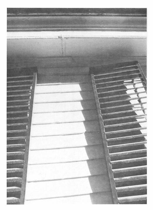
The North Front, showing the eaves where the joint between the original house and the addition of 1781 can still be seen in the joints of the mouldings under the soffit. Note the mitre joint in the mouldings which clearly shows the position of the original end wall, as this would have been the return of the moulding on to the end wall.
