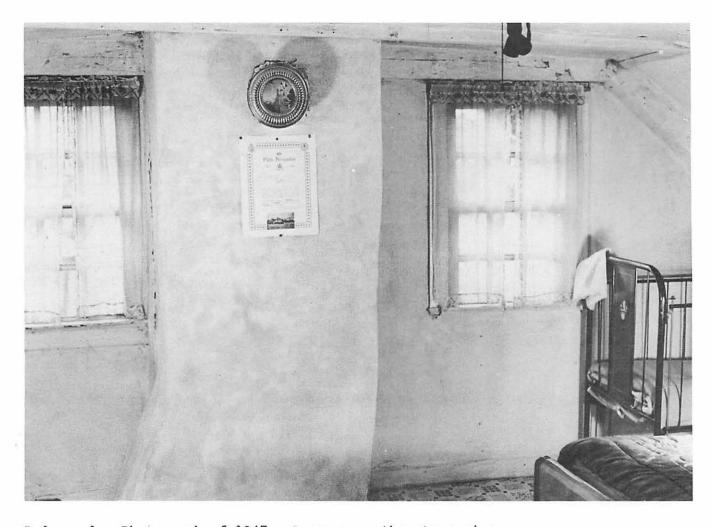
Bedroom 1. Photograph of 1947. A cap over the stove pipe connection is a reminder that Simeon Perkins poured water in here to douse a chimney fire started in the office below. This is only possible because the three fireplaces shared a common flue.
