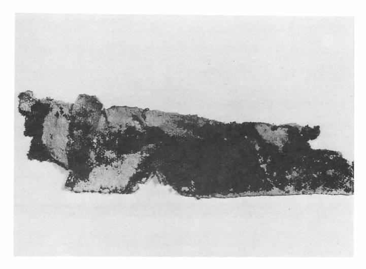
A Piece Of Canvas. Found beneath the shingles on the 1792 roof slope to the attic over the Kitchen Addition, this piece of cloth, possibly cut from an old garment, was found nailed to the sheathing under the shingles, presumably to reduce the air flow into the attic. The author found no signs of birch bark being used.
