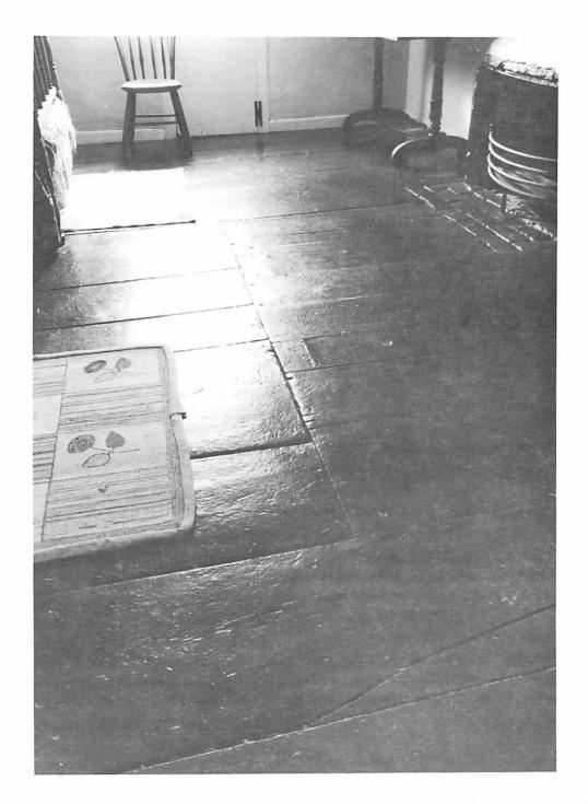
The joints in the floor boards show where the original 1767 kitchen fireplace chimney was removed. In 1781 it was rebuilt the other side of the original end wall, allowing the fireplace to merely penetrate the wall, and so provide a larger bedroom.
