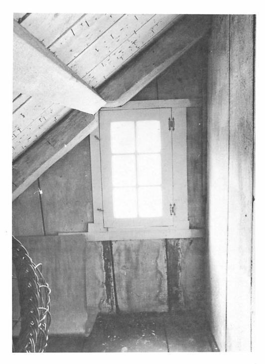
Bedroom 1 Closet looking west. Inside the closet a window opening of recent date can be seen, probably installed to improve ventilation. Note how the main rafter has been cut at the top left-hand corner to allow it to open.
