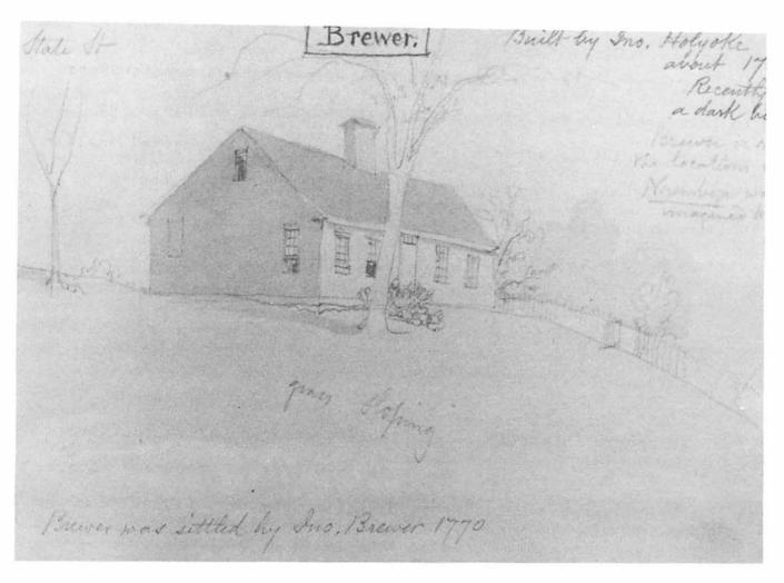
The house built by Jno. Holyoke about 1783 in Brewer, Maine. Note the symmetry of the front and the end walls, and the significantly raised centre chimney. This is the most common form of storey-and-a-half dwelling throughout New England.
