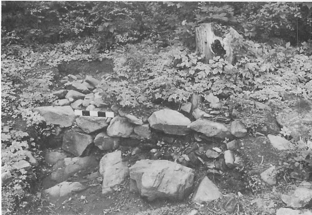
15. Haha wall, unit #8, looking west, wall face and grade fill. (See text pp.6, 8 )
