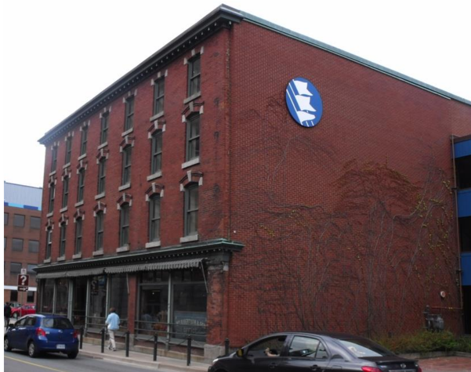
Plate 71 – Modern brick completely covers the southern stone face of the Robertson Store. Looking northeast.
