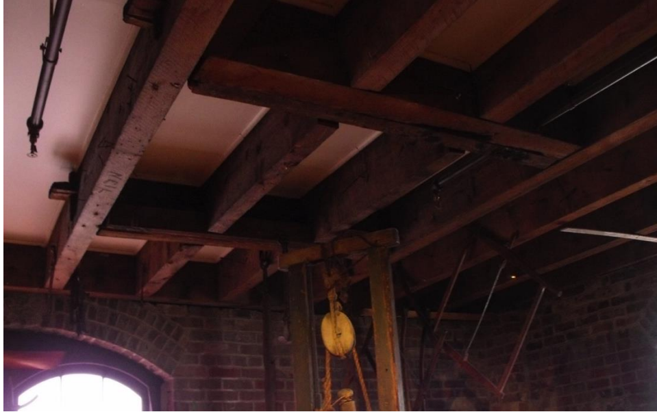
Plate 37 – A blocked hatch in the northeast corner, inside an enclosed glass display area.
