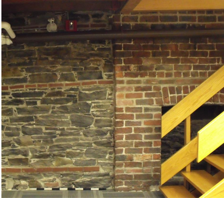
Plate 49 – The eastern end of the exposed south wall, showing new brick stringcourses and the historic brick fireplace mantle.
