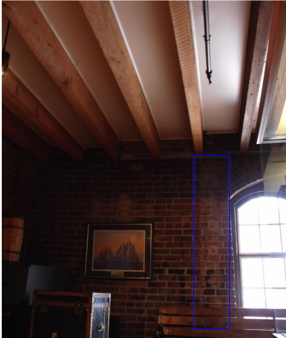
Plate 36 – Slight staining beside the window (blue) and new floor joists above clearly show where the freight elevator was located until the late 1970s. Northwest corner, looking north.
