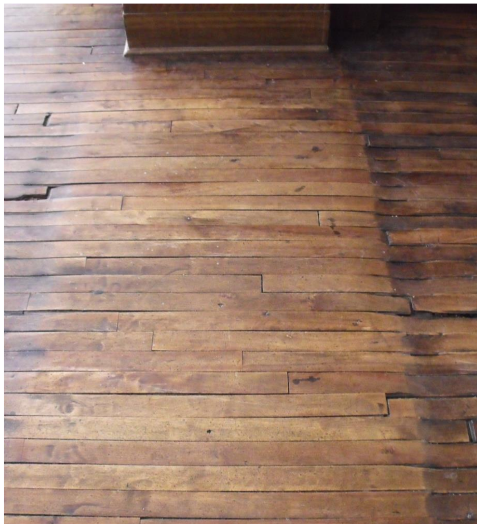
Plate 17 – Worn floorboards show the original length of the shop’s counter.
