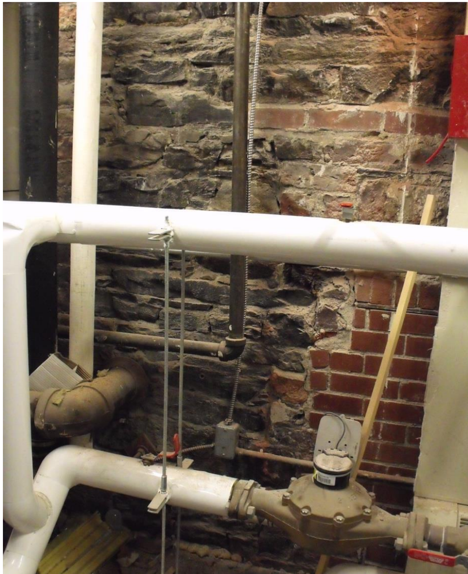
Plate 19 – The south wall of the electrical room, showing twentieth century brick repair partially behind a drywall sheet.
