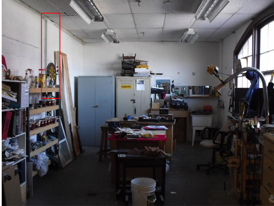
Plate 30 – The paint room, looking west. Note the boxed-in cast iron beam inside the cinderblock wall (red).
