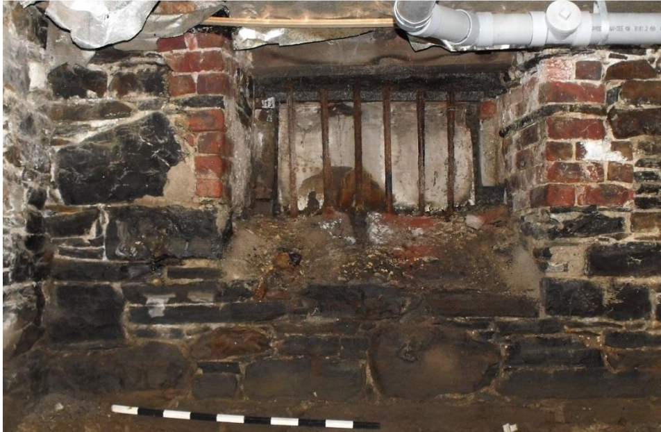
Plate 12 – The southernmost blocked window in the west wall.
