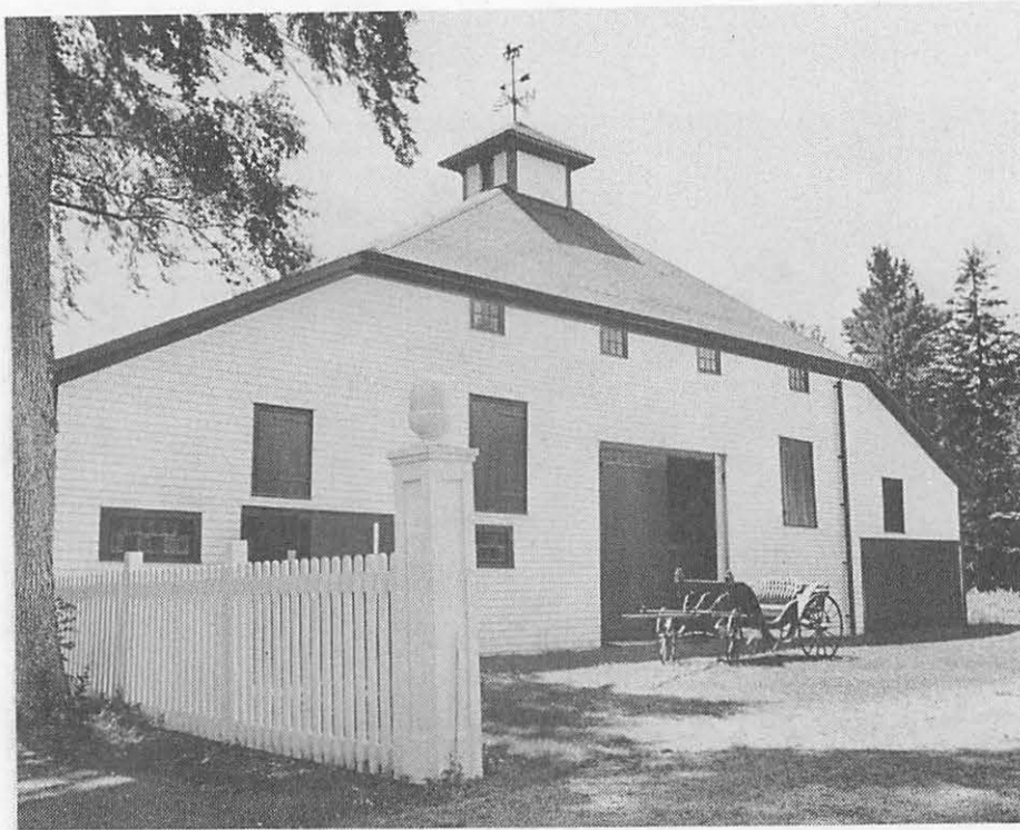
Illus. 30 The barn, as it exists today. NSM neg. N-12,423 #1 See Penney, p.32.
