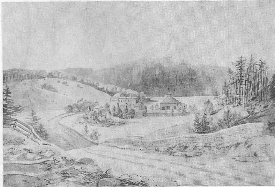
Illus. 14 "Mount Uniacke" from the Halifax-Windsor road, looking southeast, from a spot near the present - day, i.e.1991, caretaker's house. Wash drawing by John Elliott Woolford in Sketches in Nova Scotia 1817 NSM History Collection 78.45.59. NSM neg. N-8160. See Zuck, p.14; Wilson, p.20; Penney, p.31; Elwood, p.55; Gilmour, p.74.
