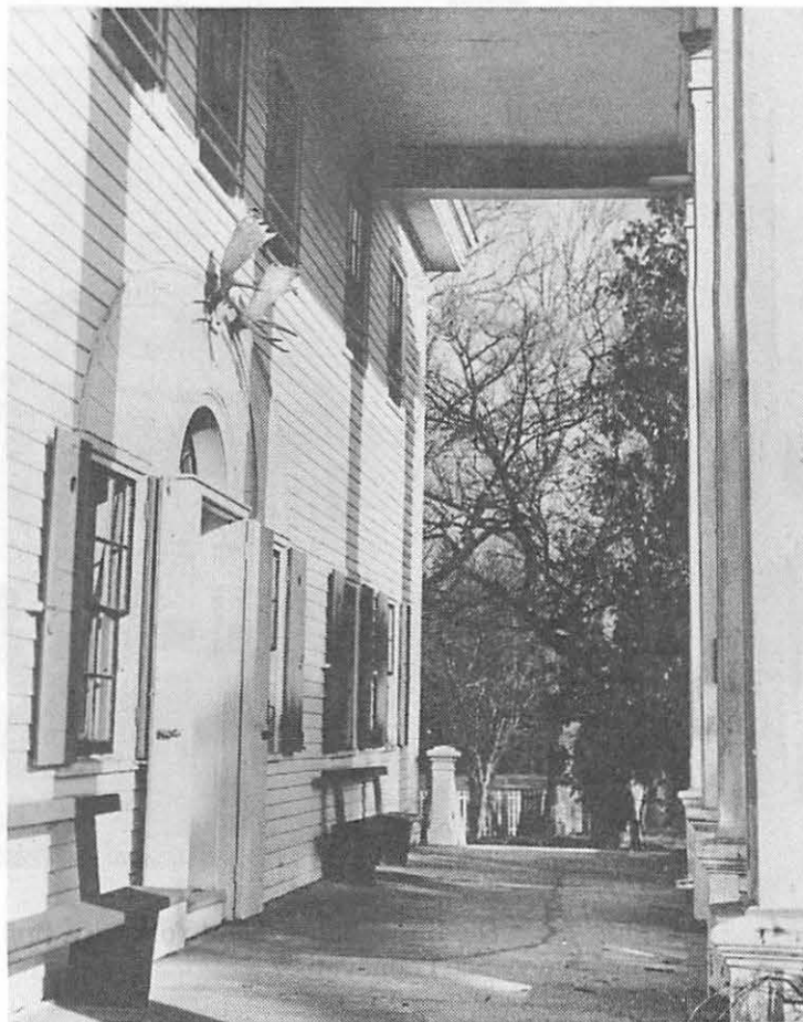
Illus. 49 Square columns and diminutive bases replaced the originals. This photograph was used as the frontispiece to K. Hale's book Historical Houses in Canada , Ryerson, 1952. Photo in NSM History Collection 71.48.2. p. 20. NSM neg. N-17,628. See Penney, p.37.
