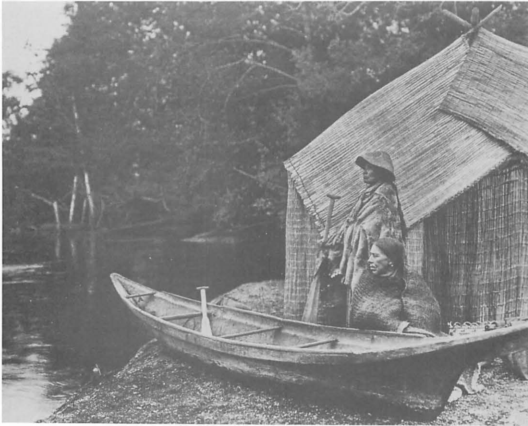
Figure 15. "Fishing Camp: Skokomish, 1912" showing a temporary summer house of cattail mats. Photo by E.S. Curtis courtesy British Columbia Archives and Records Service #74443 D-8249.
