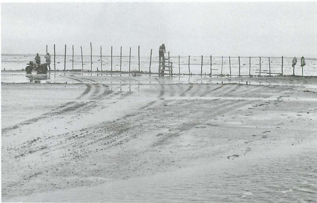
*Figure 23. The team of four men pounding the stakes for the weir.*
