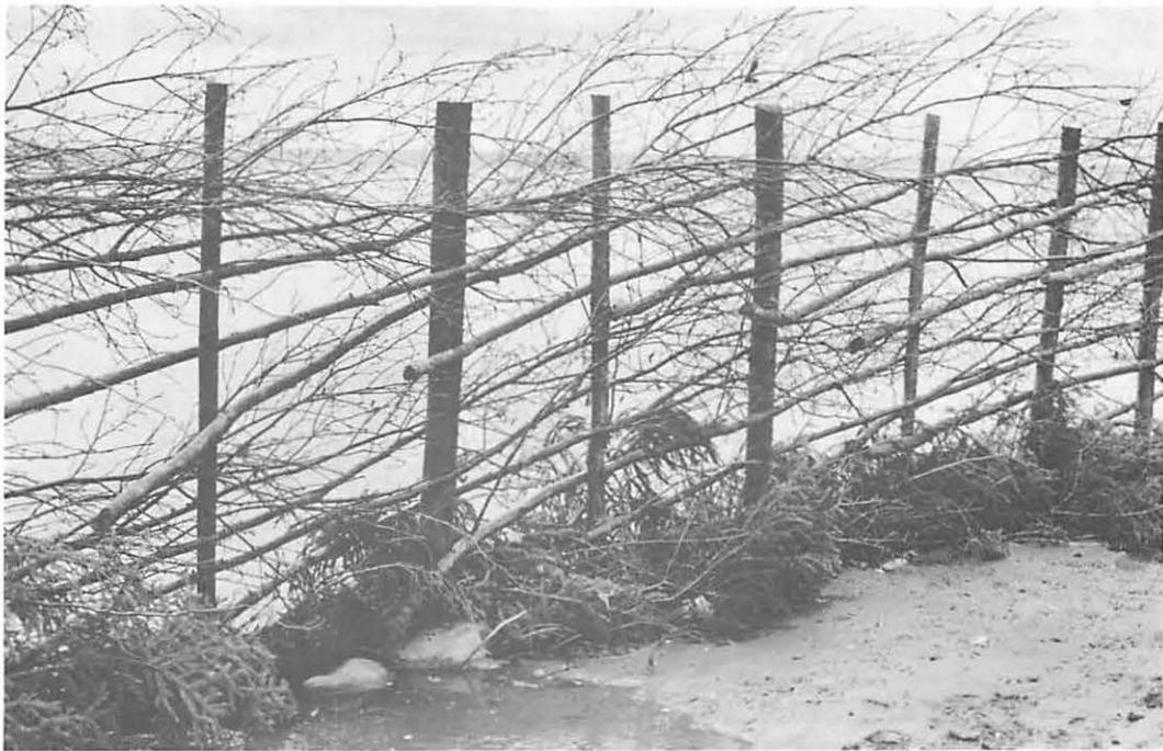
*Figure 41. Rocks are often used to fill holes between the bottom weaving and the ground.*
