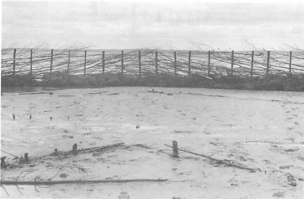
*Figure 40. The landward side of the V, showing the additional hardwood spear on the right used to fill in a space in the weaving. In the foreground are the V-stakes of an earlier weir.*
