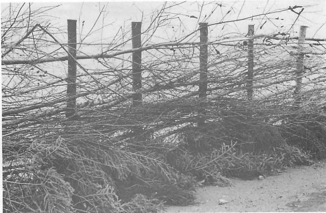
*Figure 38. In the central part of each wing, the uppermost layer of hardwood brush is woven horizontally.*
