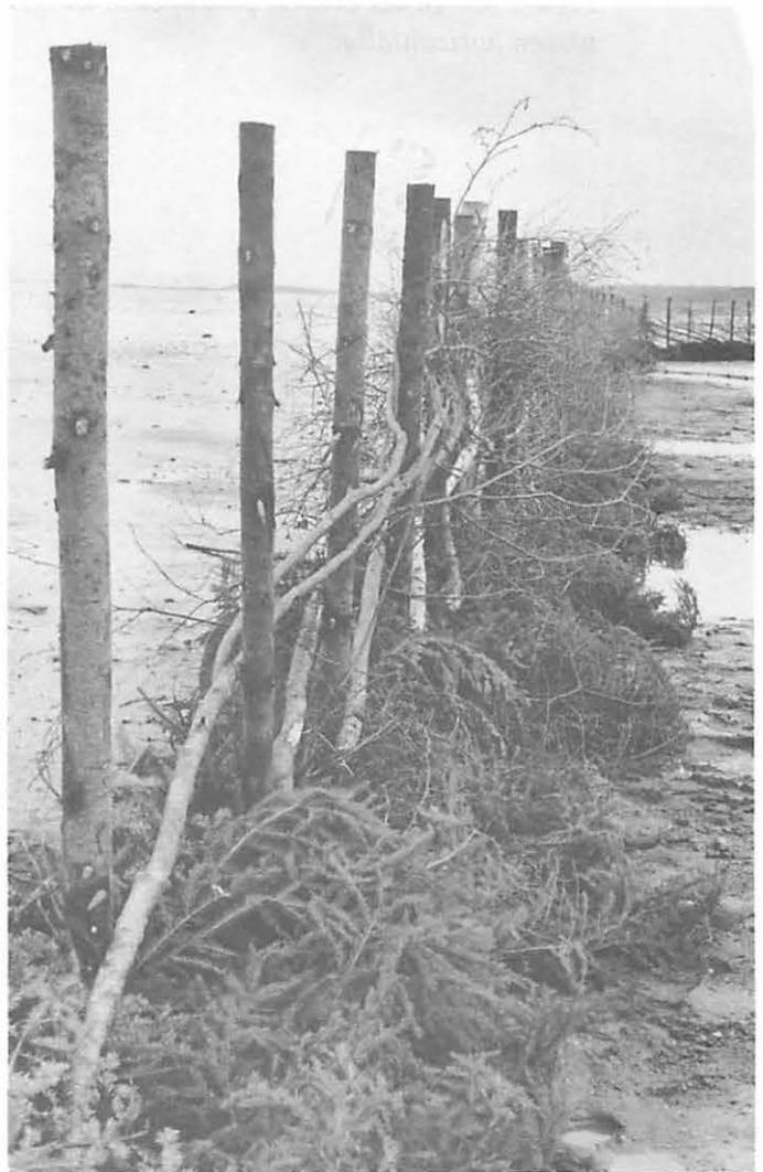
*Figure 37 On the landward side of the position in figure 25, showing the first layer of hardwood brush woven on an angle in between the stakes.*
