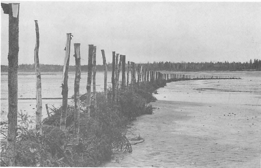
*Figure 31. The softwood brush-weaving completed all along the weir.*
