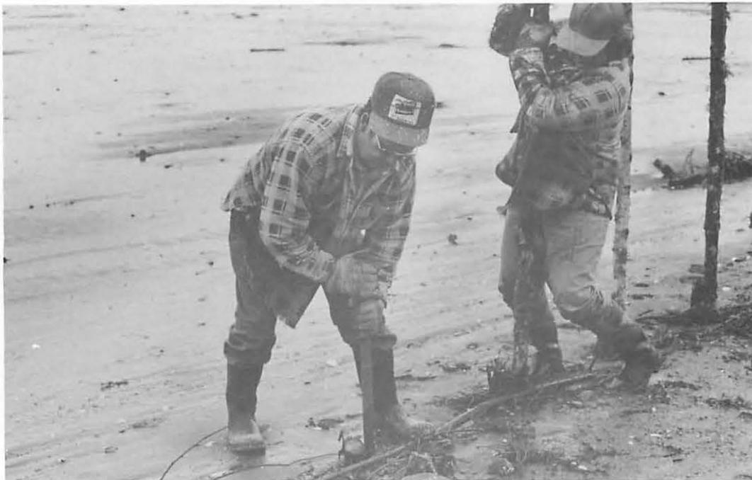
*Figure 19. James Webb, on the left, plunging the crowbar into the ground to mark the position of the next stake, while his son Todd shoves a stake deep into the previous hole.*
