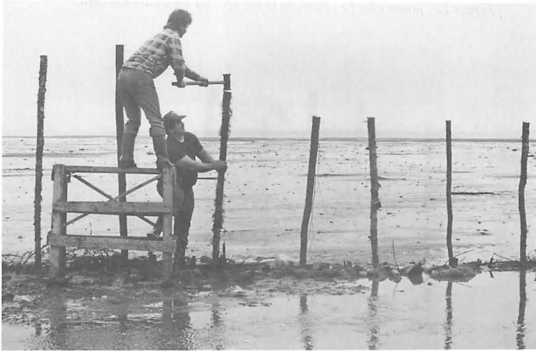
*Figure 20. Pounding the stakes firmly into place; Steven swings the maul while Jeff holds the stake in place.*
