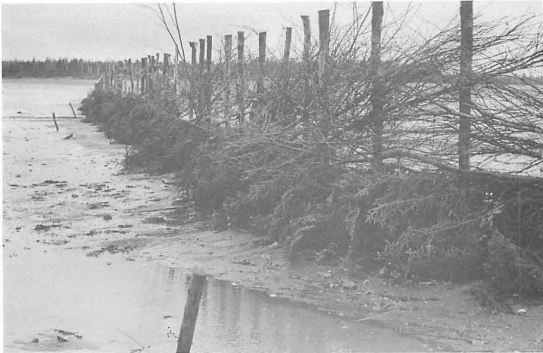
*Figure 42. The short stakes on the seaward side of the trap for the bracing lines.*
