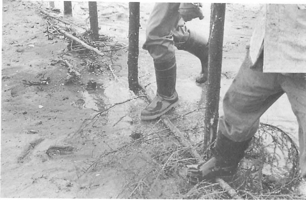
*Figure 28. Tramping the butt end of a softwood spear to the ground.*
