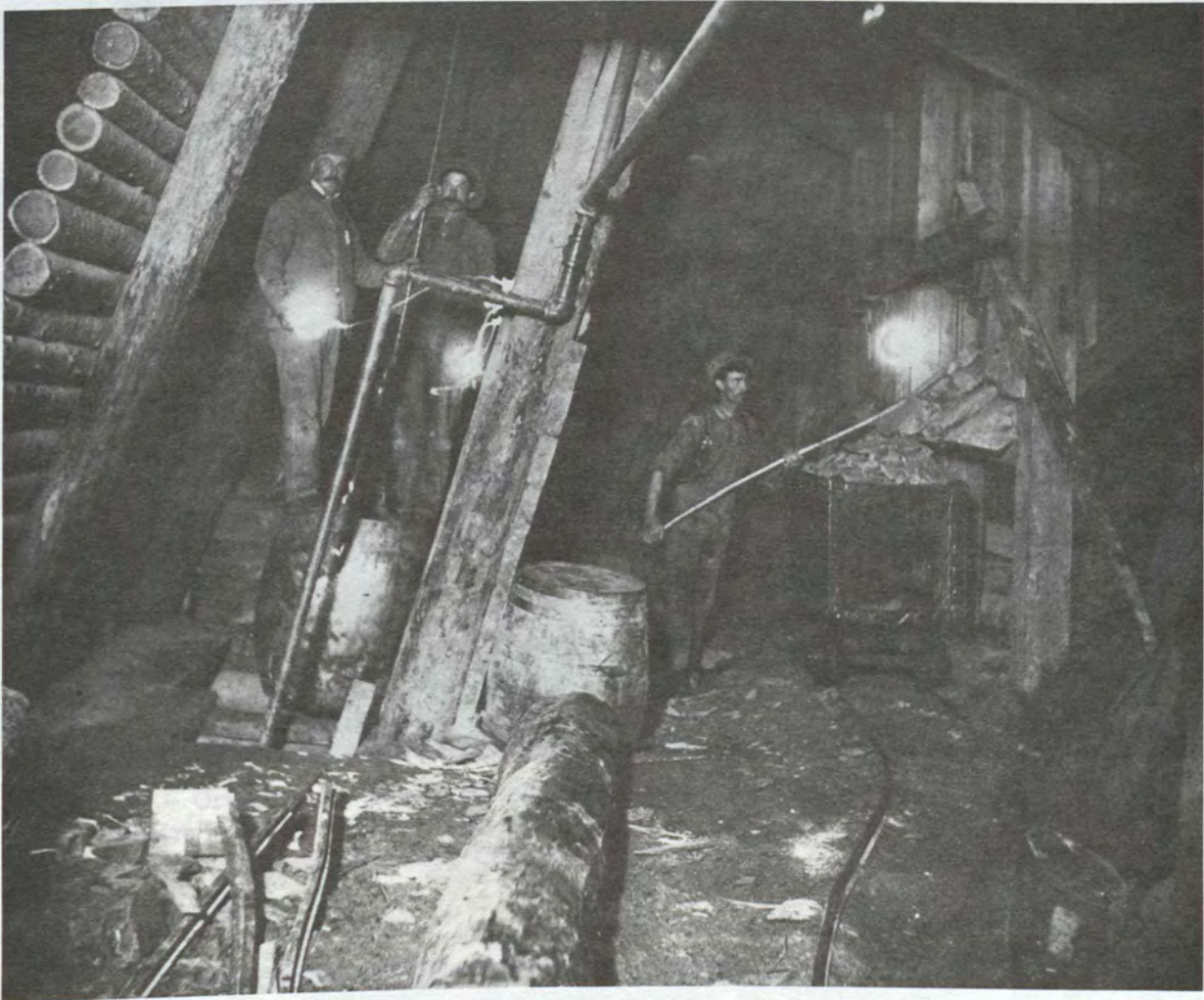
ILLUS. 33 - Ore being loaded into ore-car from chute connecting the stopes at the Baltimore and N.S. Gold Mine, Caribou, circa 1904. The man working at the ore chute would be classified as a mucker. See reference to chutes on page 69, this report. NSM N-5193.
