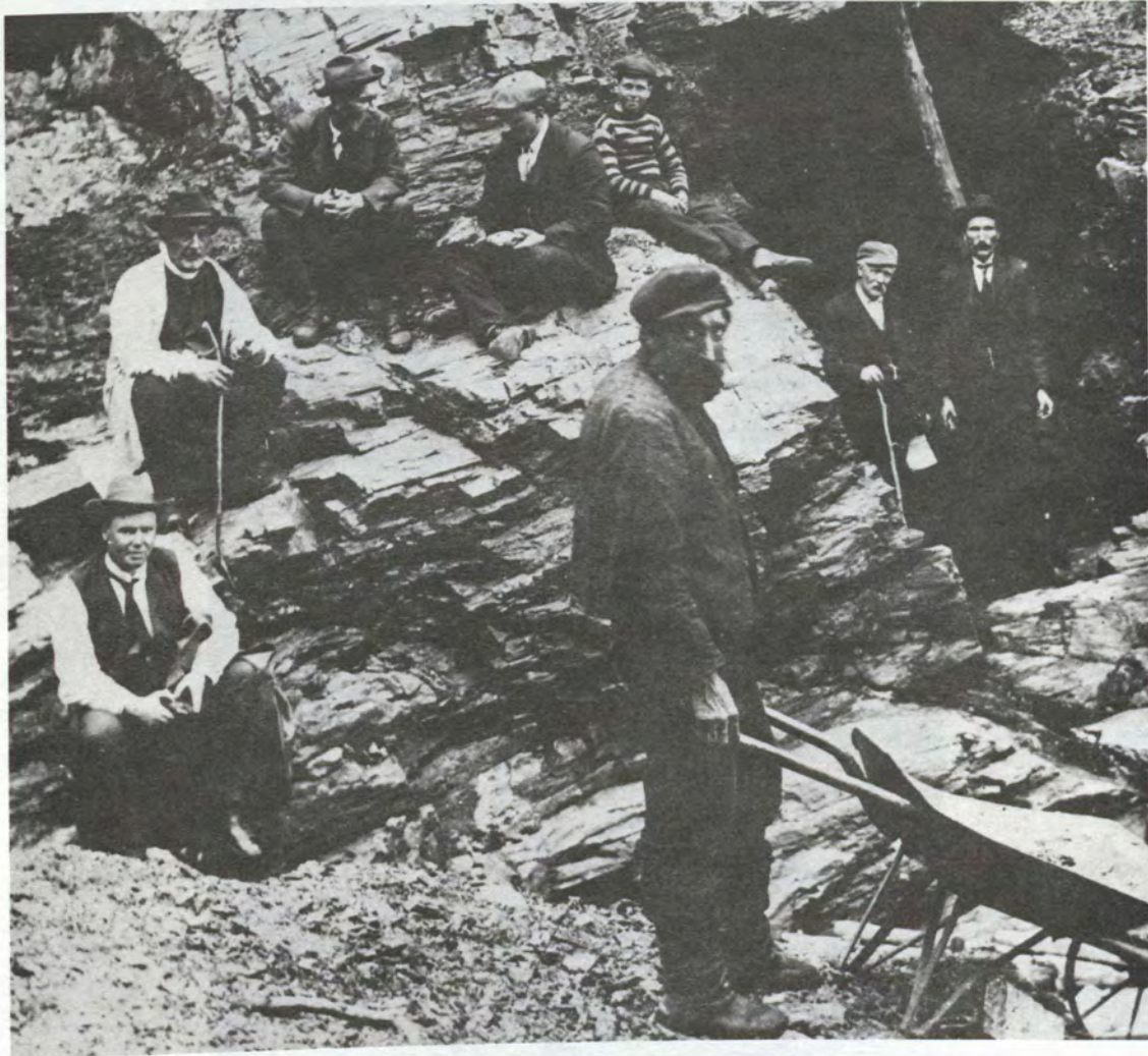
ILLUS. 38 - Unidentified tunnel. NSM N-2650.
