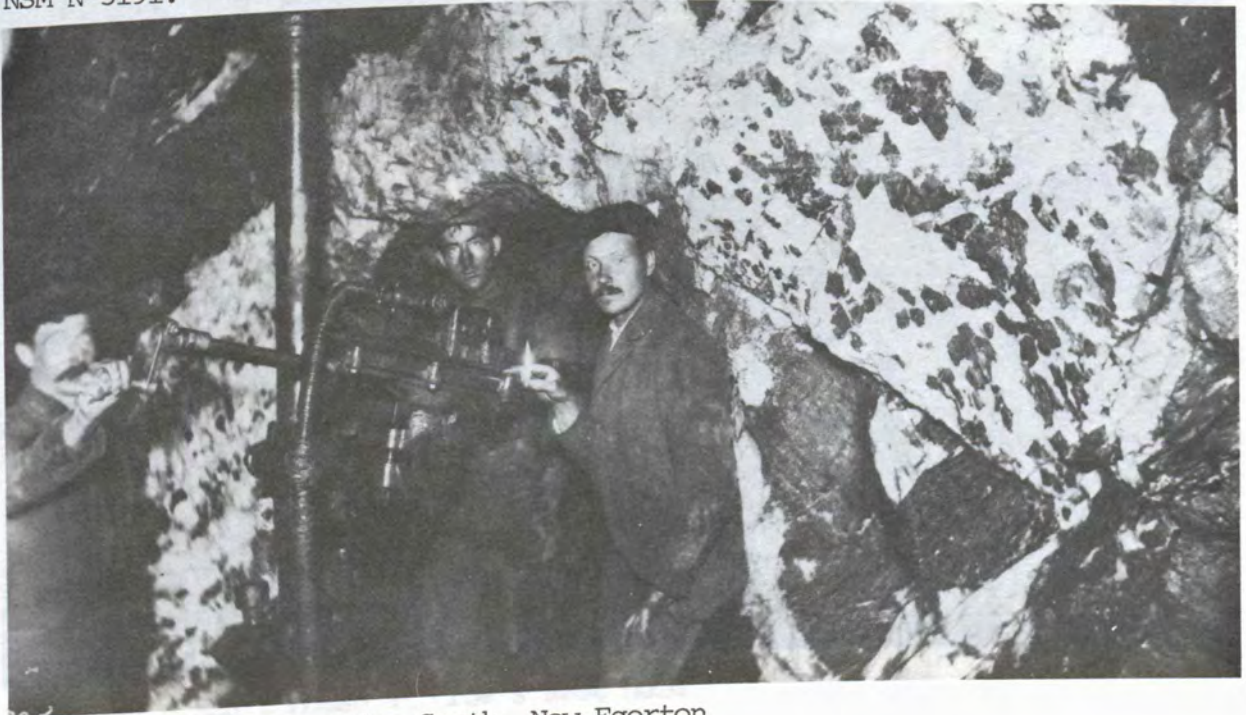
ILLUS. 45 - Cross-cutting South, New Egerton Gold Mining Company, Fifteen Mile Stream, using early air drill, 1897. Candle-power provided the light. PAC 39894.
