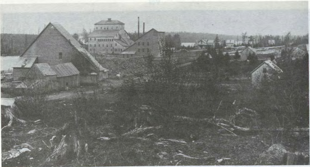
ILLUS. 54 - Shaft house and mill. Baltimore and N.S. Mining Co., circa 1904. NSM N-9780. The power source is housed at ground level also at some distance, if not separately, from the mill.
