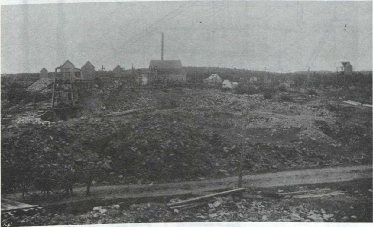
ILLUS. 48 - New Glasgow Gold Mining Co., Goldenville, 1897, looking east. Shaft houses. PAC 39882.
