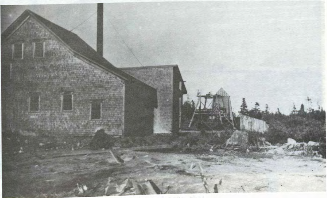
ILLUS. 53 - Harrigan Gold Mine, 1893. Mill building. PAC 39830.
