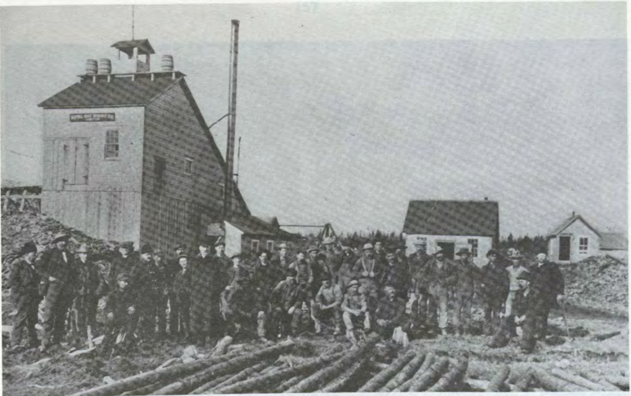
ILLUS. 50 - Power house and shaft. Royal Oak Mine, Goldenville, 1902. Windows provided natural light. Engine and boiler were located on the ground level. NSM N-10519.
