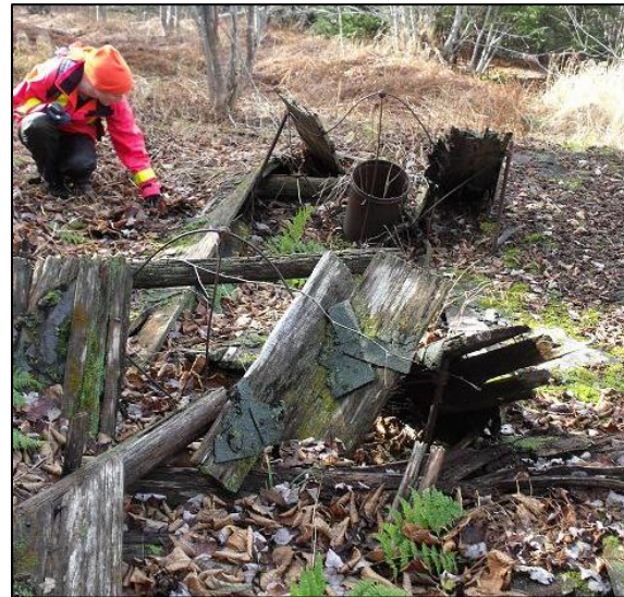
Plate 2: Cast iron bed frame protruding from the cabin collapse.
