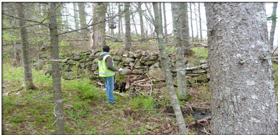
Plate 1: Surveying the retaining wall.
