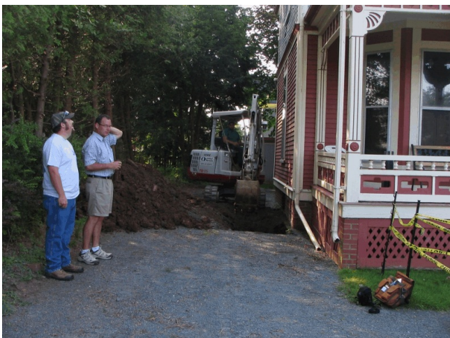
Plate 1: Trench excavation on eastern (driveway) side of Shand House.
