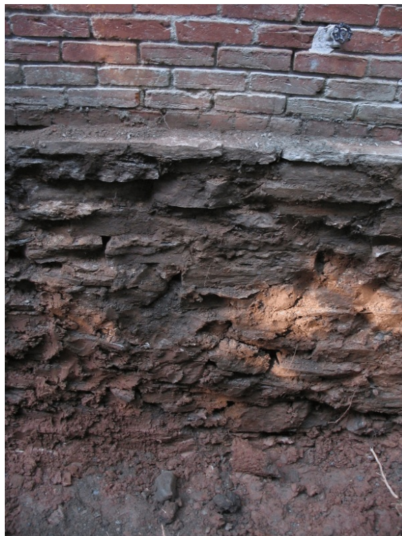
Plate 3 - Dry stone foundation below brick is resting on natural reddish clay.
