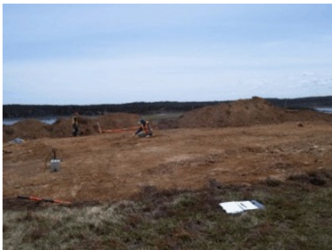
Plate 1: Manual excavation around the ground shafts after the overburden has been mechanically removed.
