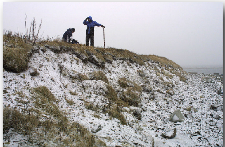
Recording coastal change at a survey marker located on the Louisbourg coastline. © Parks Canada Agency
