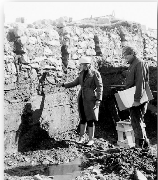
Mooring rings in Louisbourg quay wall ©Parks Canada Agency
