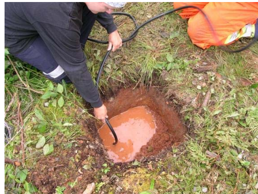
A pump hose removes water from a test pit in Debert. (K. Cottreau-Robins, 2011)
