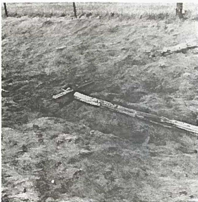
Figure 5. Abandoned telephone pole with four pin crossarm in a roadside ditch at Amherst Shore, Cumberland County.
