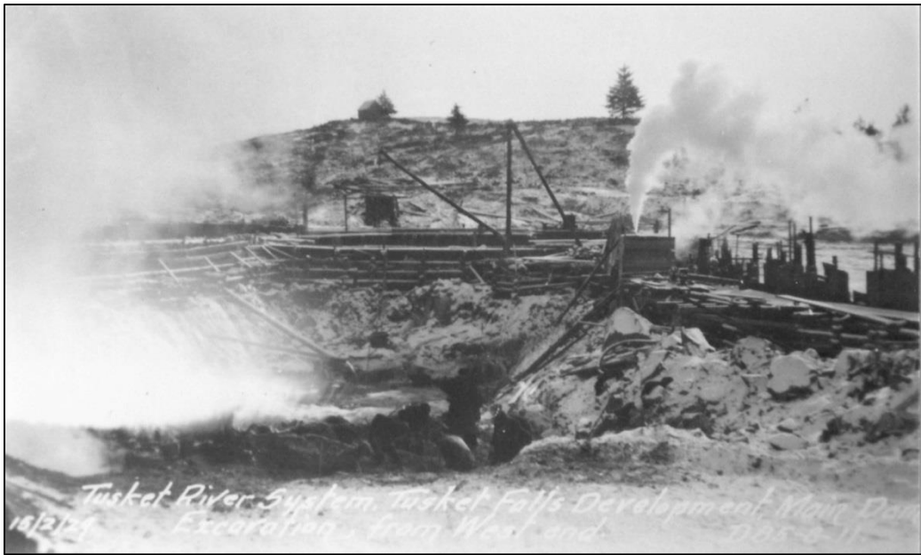
Plate 11: Excavation of the main dam in 1929 with steam powered Errie shovels (Argyle Township Court House Archives P1999-712pf).
