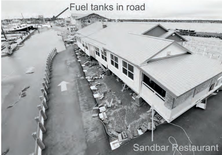
Fig 1 The Pointe-du-Chêne Wharf, NB, on 24 September 2022, a few hours after the passage of Fiona. Note the Sandbar Restaurant that was pushed off its foundation (which also happened during Hurricane Dorian in 2019) and the wharf's fuel tanks that were pushed into the road. Photo credit: Andrew Ollerhead.
