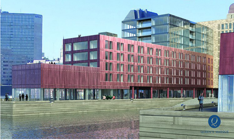
Fig 5 Architectural concept drawing of the south building of the Queens Marque development that is presently under construction on the Halifax Harbour waterfront. Note the stilt design of the ground floor (source: https://my-waterfront.ca/development/queens-marque ).
