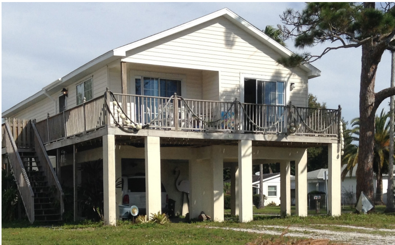
Fig 4 Stilt homes featuring ground level storage and 2 nd floor living areas are becoming more common in coastal and flood prone areas of many southern states (e.g., Florida) (Photograph by author).
