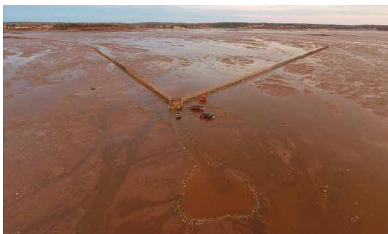
Fig 12 The Bramber weir at low tide in Minas Basin that was used for the 2017 weir study (Dadswell et al. 2020). The v-shaped wings direct fish into the trap at the bottom of the photograph. Fisher’s trucks are clustered around the trap. The channel leading from the trap and heart shaped structure (pond) is where fishes prohibited from take (sturgeon, striped bass, salmon) are released alive to await the return of the tide (photograph courtesy D. Porter, Avondale, NS).
