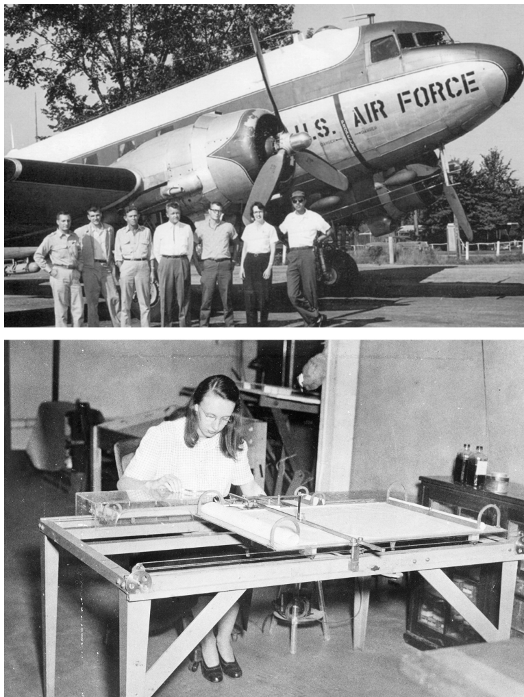
Fig 4 Elizabeth King working among the crew of the aerial survey group of the United States Geological Survey c.1956 (above), and working a graph rectifier (USGS 1952), a machine to get the continuous magnetic reading into usable form (below).
